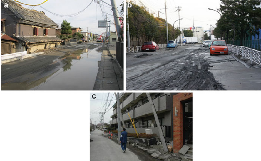
Fig. 8.5 Pictures showing damage from liquefaction in Chiba and Tokyo Bay regions (a) Abiko (b) Shinkiba (c) Urayasu
