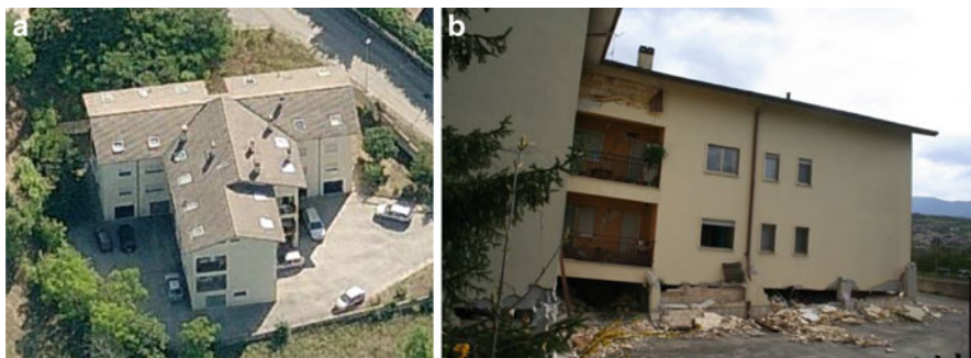
Fig. 10.7 (a) Pre-event view of case study building, placed in Pettino (L'Aquila) (from Virtual Earth); (b). Collapsed building (Verderame et al. 2011)
