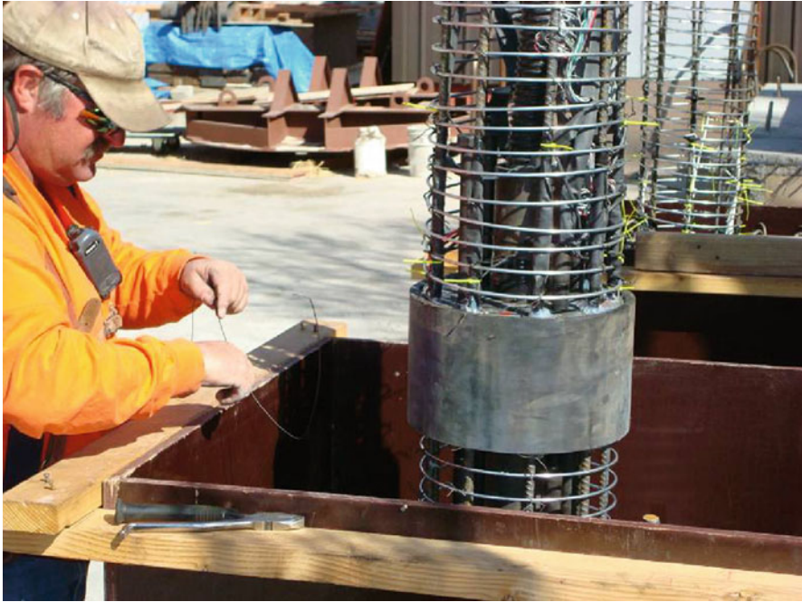
Fig. 5.4 Elastomeric plastic hinge embedded in the column cage
