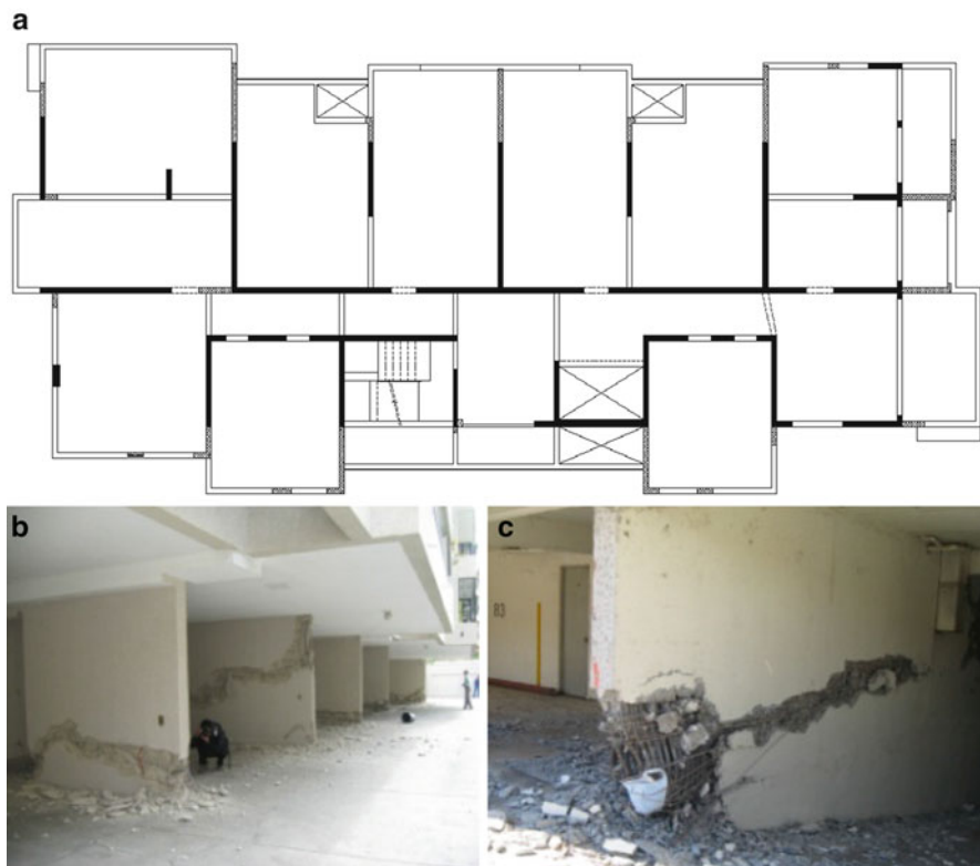
Fig. 11.5 (a) Typical plant of R/C wall building in Chile, (b) Typical failures in R/C walls, localization caused by buckling of vertical reinforcement, and (c) Buckling of bars in a boundary element
