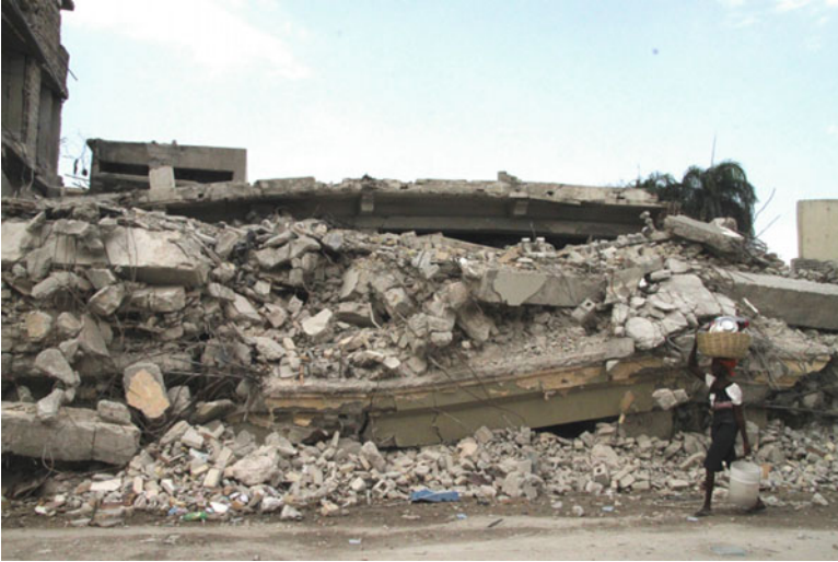
Fig. 9.6 Complete collapsed building in downtown Port-au-Prince
