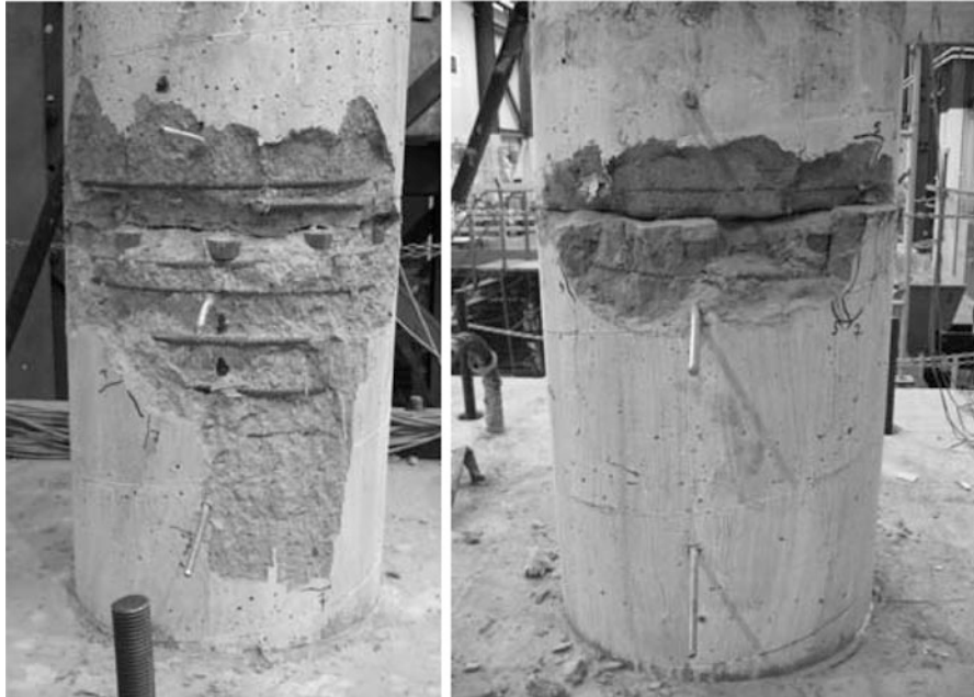
Fig. 5.7 Damage at RC (left) and ECC (right) plastic hinges of segmental columns
