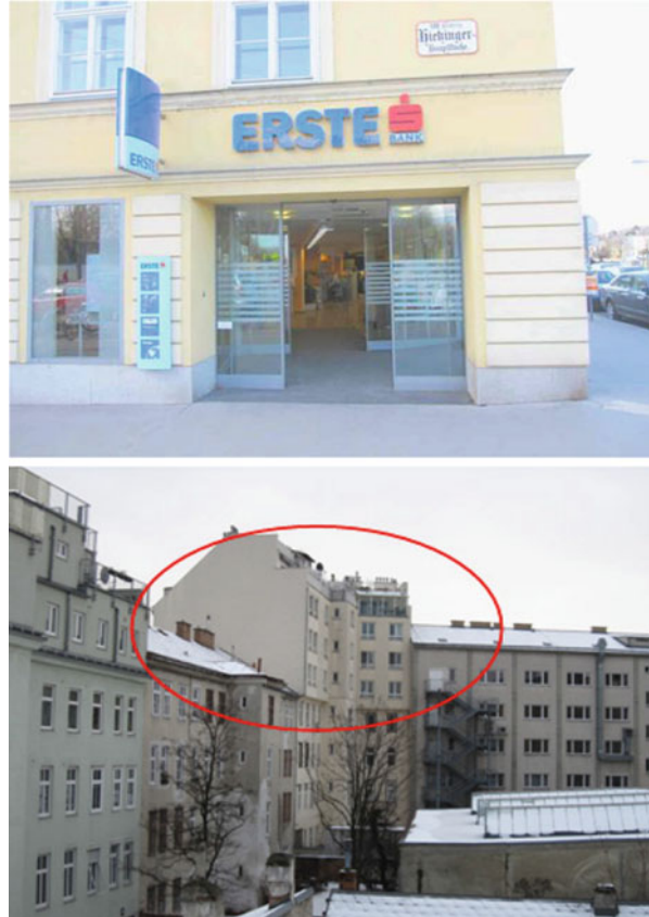
Fig. 8.8 Identifying soft stories and additional attic spaces
