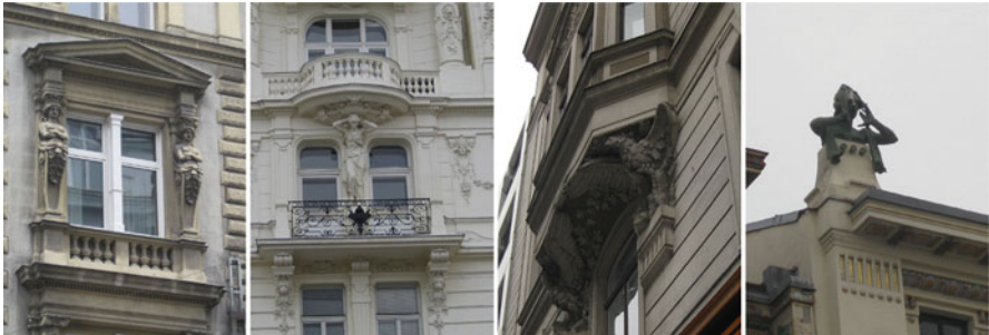
Fig. 8.11 Examples for non-structural members
