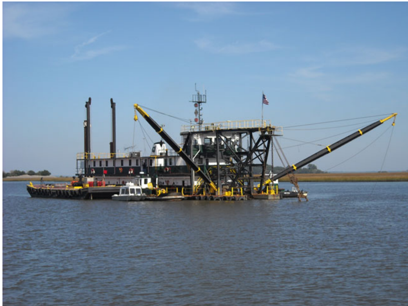
Dredging, Figure 1 Cutterhead dredge, with spuds deployed at rear, and cutterhead suspended from opposite end.
