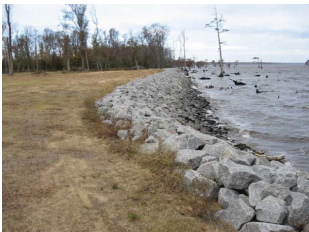
Coastal Erosion Control, Figure 11 Rip-rap revetments (Trowell, 2012).
