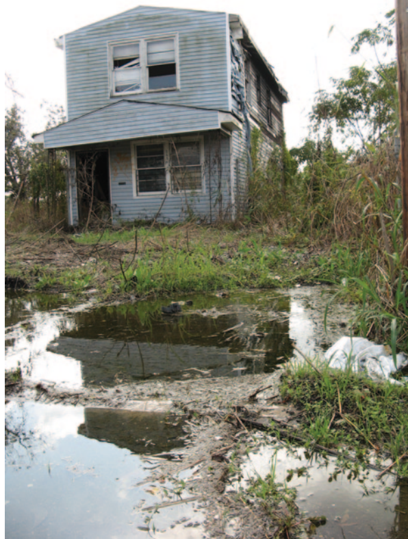
Fig. 15.3 Derelict house, Lower 9th Ward, New Orleans. (Source: photograph by Bruce Glavovic)
