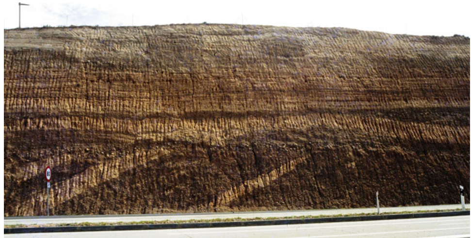
Fig. 9.6 Cutting of the Madrid–Zaragoza highway (A–2) next to Calatayud Hospital, showing a non-tectonic angular unconformity between dipping alluvium of terrace T8 and subhorizontal deposits of terrace T4
