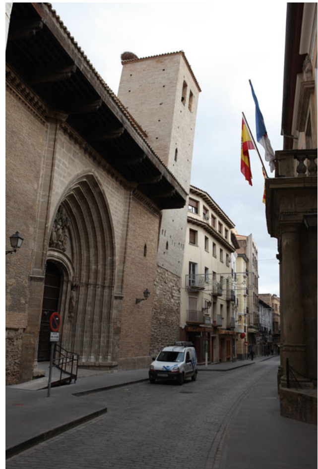
Fig. 9.9 Tilted tower (11th–12th C) of San Pedro de los Francos Church (14th C) in La Rúa Street. The upper 5-m-high portion of the tower was removed in 1840 to avoid its collapse over the Wersage Palace located in the opposite side of the street, where the Royal family used to be hosted
