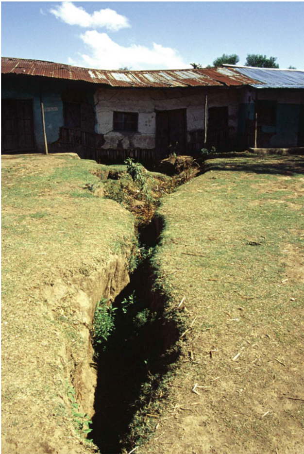
Fig. 20.7 House damaged by a ground fissure at Meki (Photograph by V. Acocella)
