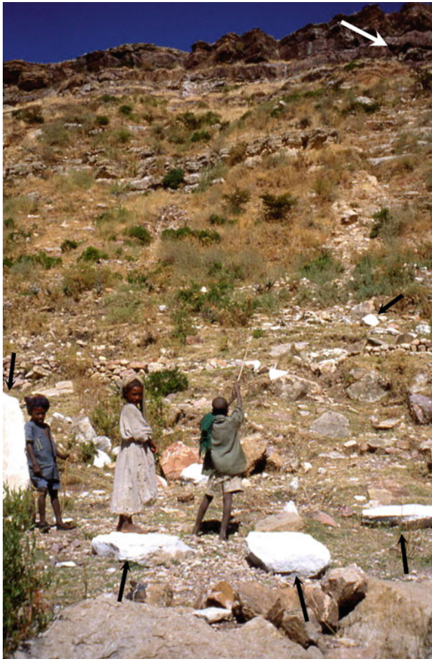
Fig. 9.5 Three months after the occurrence of a rockfall event (August 1998) on the sandstone cliff. Fresh rock fragments ( arrows ) are easily recognisable by their bright colour. The upper arrow indicates the place of origin of these rocks on the cliff. Despite recovering vegetation, the rockfall path can still be recognised on the backslope (after Nyssen et al. 2006)
