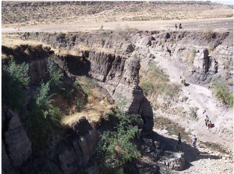
Fig. 11.8 Toppling affecting the Mai Makdem tufa dam backfill
