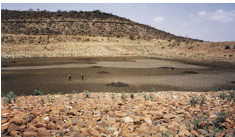
Fig. 13.6 Part of the layout of the 26 profile pits at Gereb Shegel reservoir where sediment deposits are up to 3 m thick near the dam (left) and details of topographic mapping and sediment profile pit layout
