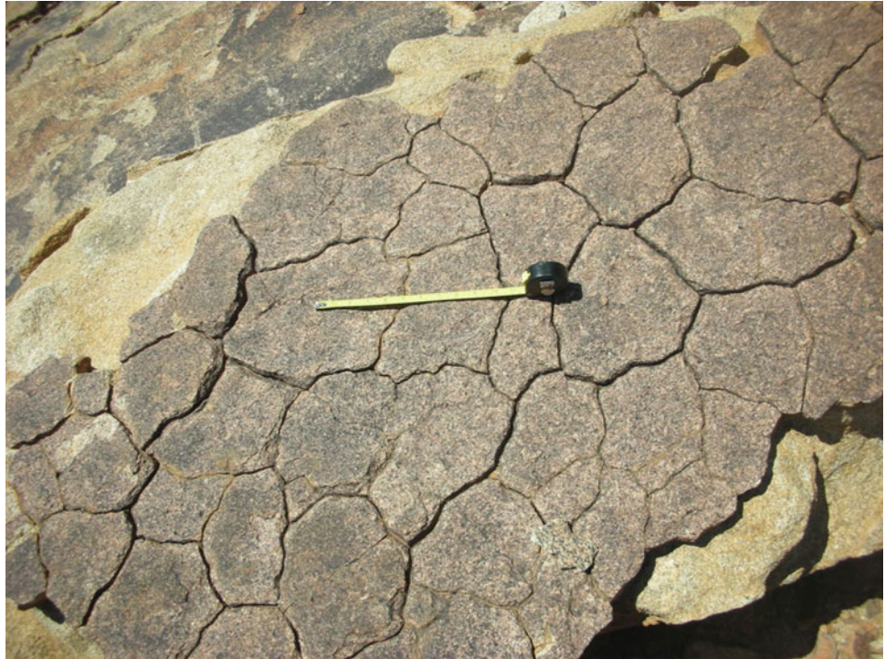
Fig. 11.5 Polygonal cracking in granite, Phillip's Cave
