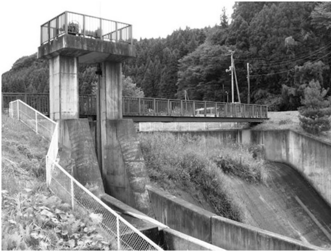
Fig. 9.13 Location of sampling site in concrete canal (Photo Head works)
