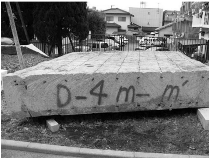
Fig. 9.10 Concrete arch member of the Gion Bridge
