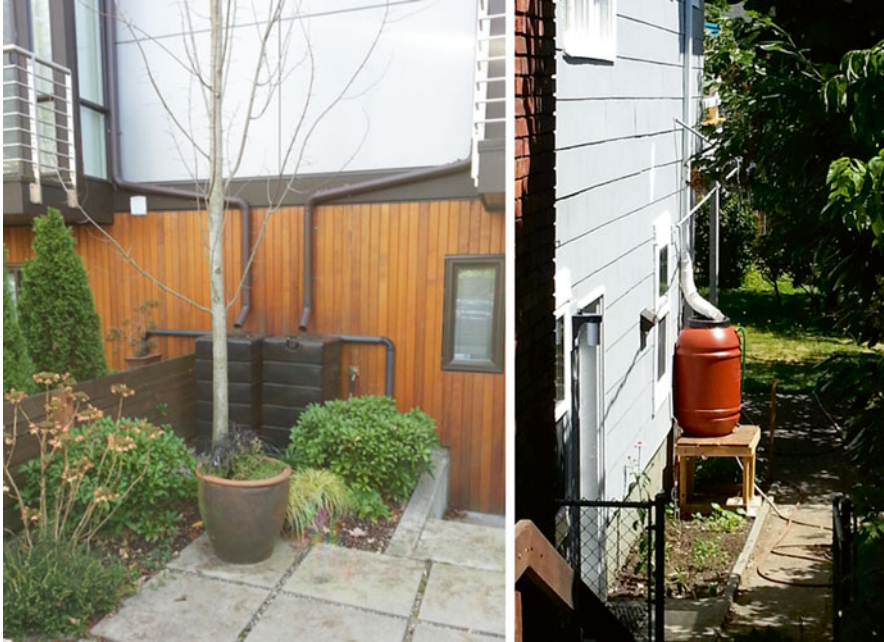
Fig. 1 Stormwater collection barrels in Seattle, WA. The newer home was designed to include a stormwater barrel while at the older home, the owners added the barrel. Seattle Public Utilities sells and delivers rain barrels to customers ( http://www.seattle.gov/util/environmentconservation/mylawngarden/rain_water_harvesting/buyrainbarrels/ )
