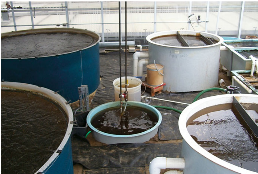
Fig. 6 Production tanks, sump tank, solids filters – An important part of any aquaponic system is a series of filters to remove the suspended particles from the water (solids filter) and to convert the ammonia excreted by the fish to nitrate nitrogen (biofilter). This picture contains the production tanks on the left and the solids filters on the right . In the center , is the heated sump tank where the water flowed into after leaving the hydroponic troughs. From here, the water was lifted into the production tanks using a high efficiency pump
