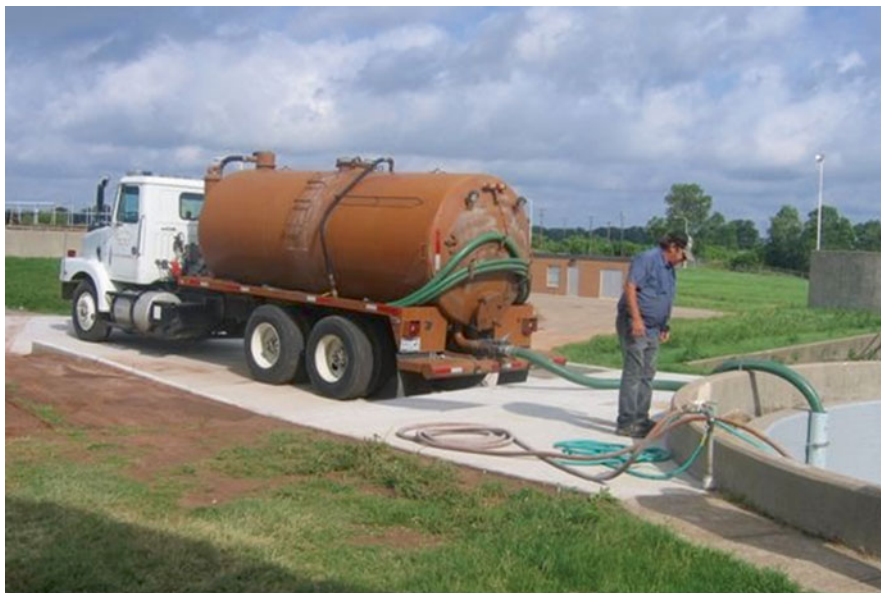
Fig. 2 High strength organic wastes from food processing being delivered to a wastewater treatment plant for direct anaerobic digestion (Photo from Michael Jupe, Waco, TX)
