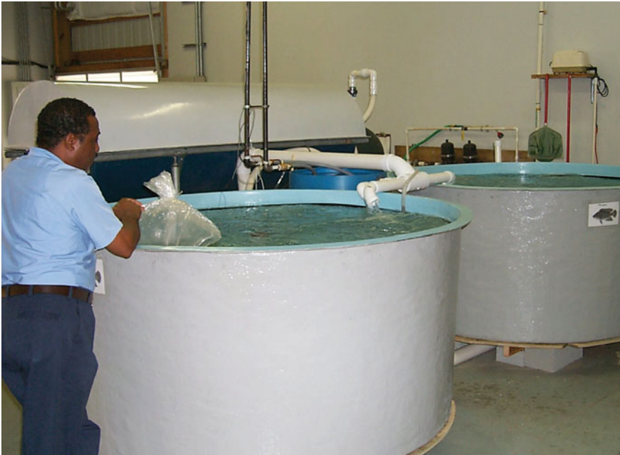
Fig. 2 Nursery Tanks – The aquaponic system at the Rutgers EcoComplex had two 600 gallon tanks for rearing the fingerlings for the first 12 weeks. This system had a separate floating bead solids filter and biofilter and was not connected to the hydroponic system. The entire system was based on the outdoor system designed and operated by Dr. Jim Rakocy and his research team at the University of the US Virgin Islands, St Croix Research Station and modified for use in the greenhouse
