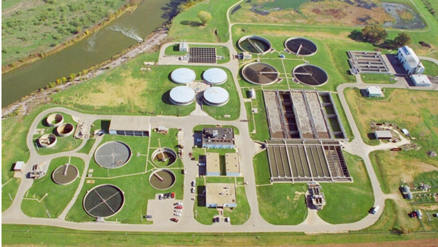
Fig. 1 The Waco Metropolitan Area Regional Sewerage System (WMARSS) Wastewater Treatment Plant (WWTP) serving the City of Waco, TX. The plant uses aerated secondary treatment and anaerobic digestion to stabilize wastewater (Photo from Michael Jupe)
