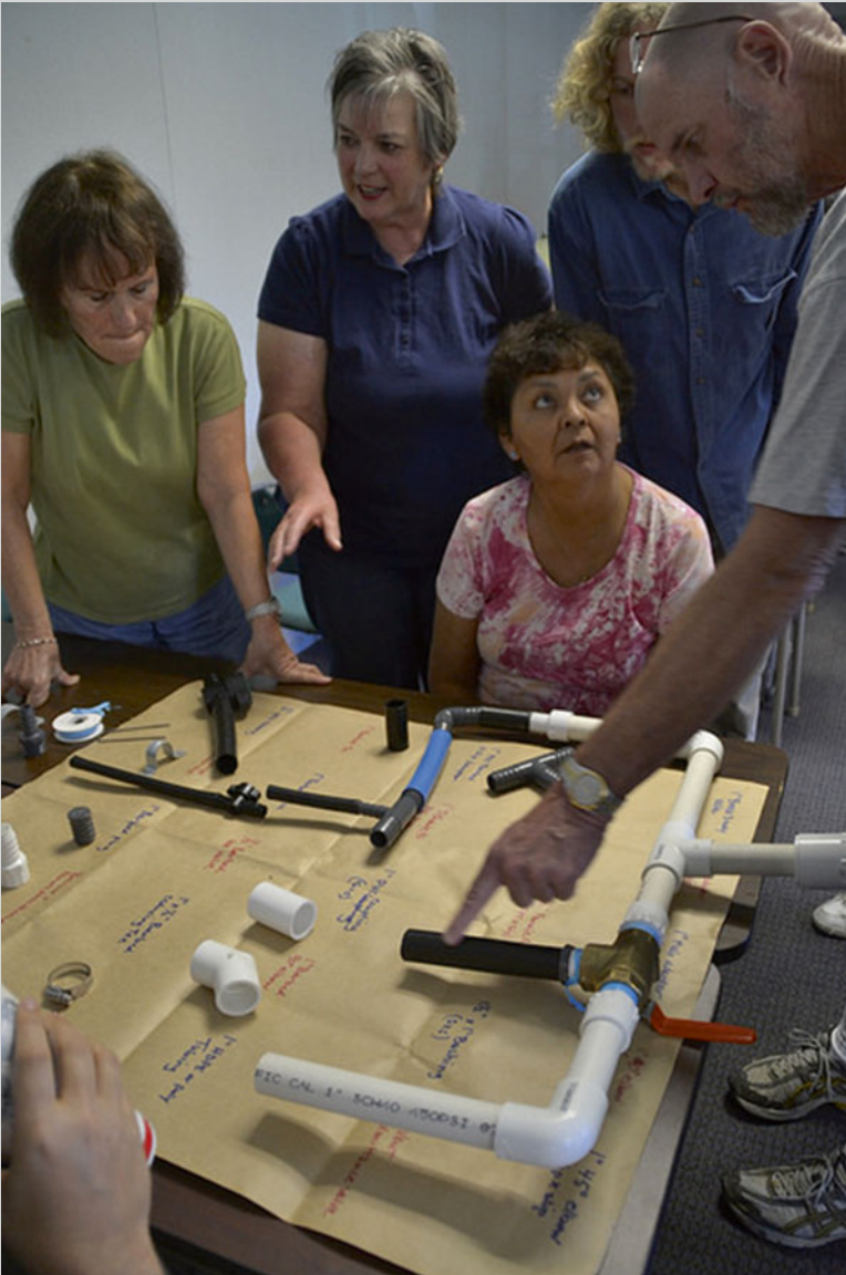
Fig. 3 A greywater workshop hosted by Daily Acts. The pictures show an indoor demonstration of the plumbing retrofit required, changing the plumbing on a washing machine, and installing the irrigation system outside a home (Photos Daily Acts)
