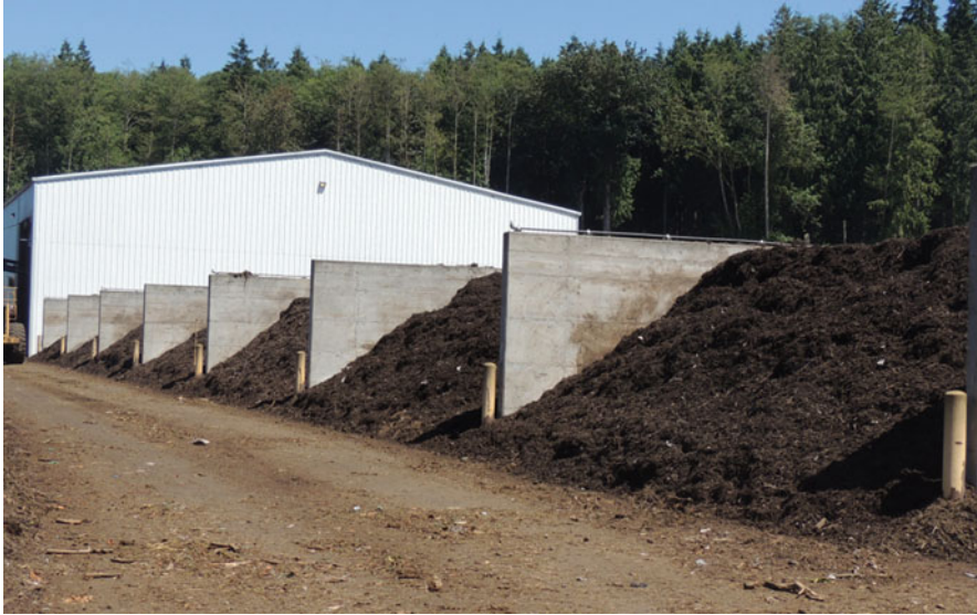
Fig. 2 Co-composting composting food and yard waste at the Lenz Enterprises compost facility north of Seattle, Washington
