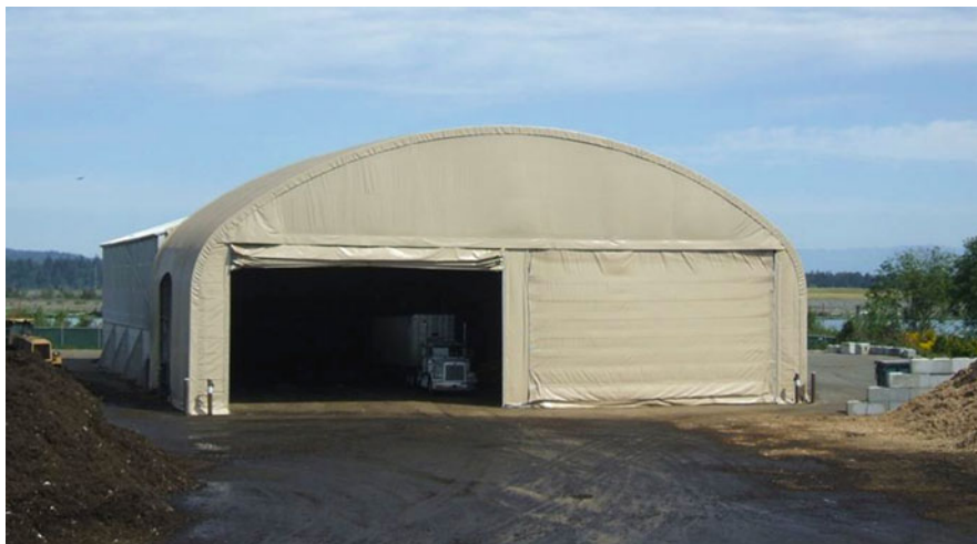
Fig. 7 The receiving building at the Everett compost facility. Enclosing the receiving area was done as a way to mitigate odors. Delivery of feedstocks is the greatest source of odor at our facility
