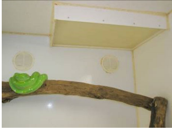
Fig. 5 Radiant heat panel
