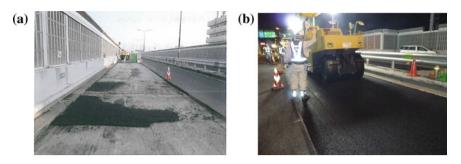
Fig. 9 Picture of construction: a repaired rough surface area, b compaction
