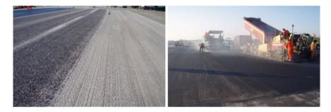
Fig. 6 SAMI section (left) and trial field completion with PmB wearing course (right)
