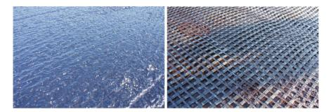
Fig. 5 PmB emulsion section (left) and fiberglass grid section (right)
