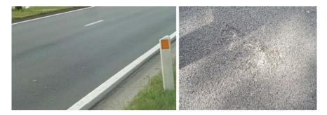
Fig. 9 Ravelling observed in test sections on the N19 Turnhout-Kasterlee
