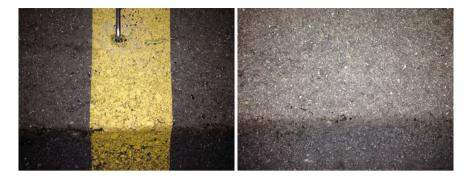
Fig. 11 HMA deterioration outside trafficked area in Test Strip-2
