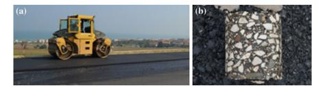
Fig. 8 In-field validation: a compaction of the recycled layer, b extracted core
