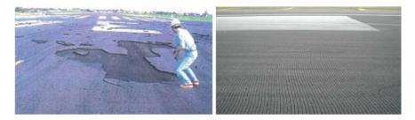
Fig. 1 Nagoya airport debonding failure and high-speed taxi way slippage
