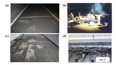
Fig. 3 Picture of conventional method: a injured surface, b gussasphalt is constructed by human power, c formation level is uneven, d PM-N was not set on flat
