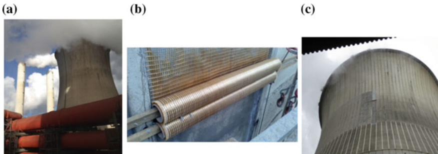
Fig. 9.1. Structural retrofitting of cooling towers with PBO-FRCM (by Ruredil): a Power plant cooling tower. b and c application of the FRCM composite
