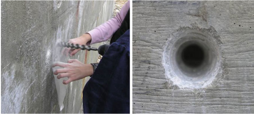
Fig. 4.35 Drilling concrete dust specimens for chloride profiling
