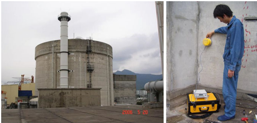
Fig. 8.26 Testing concrete quality with Autoclam in Dayawan nuclear power station by Central Research Institute for Buildings and Construction
