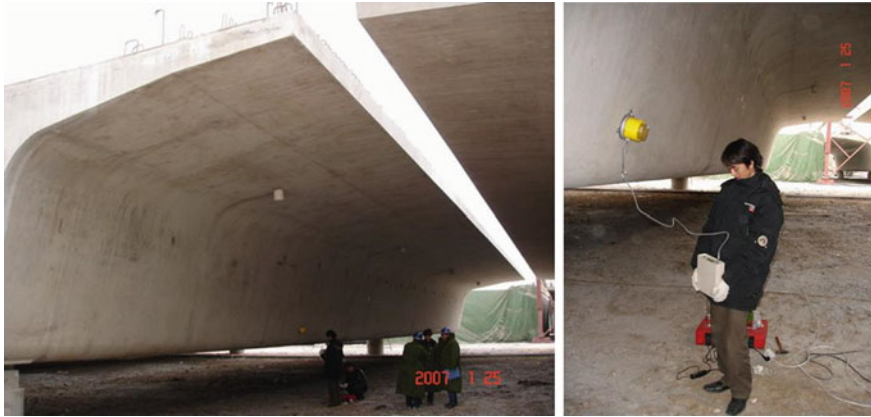
Fig. 8.28 Testing concrete quality with Autoclam in Beijing-Tianjin railway project by Central Research Institute for Buildings and Construction
