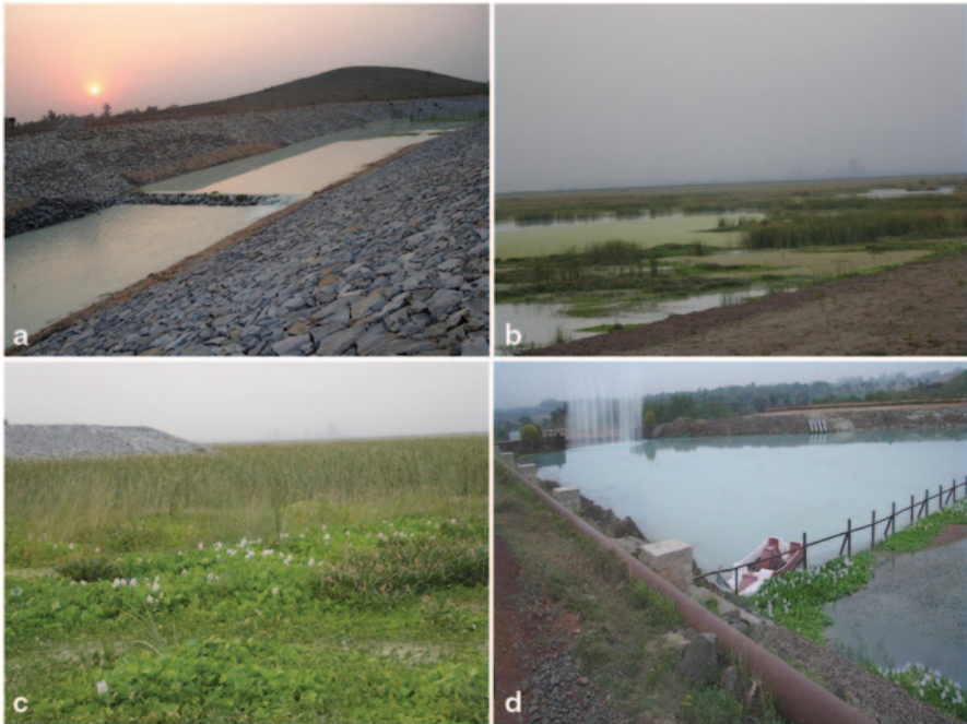
Fig. 3.12 a and b Granite lined canal discharging ash slurry water to large lagoons. c and d Constructed wetland with its plant assemblage involved in treatment of the contaminants. Cleaned water is discharged into storage pond for reuse
