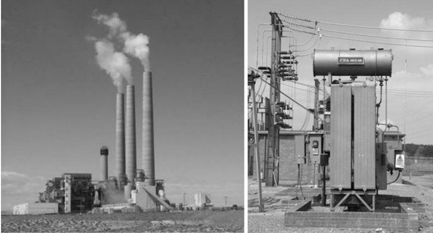
Fig. 6.1 Power-plant ( left ) and high voltage transformer ( right )
