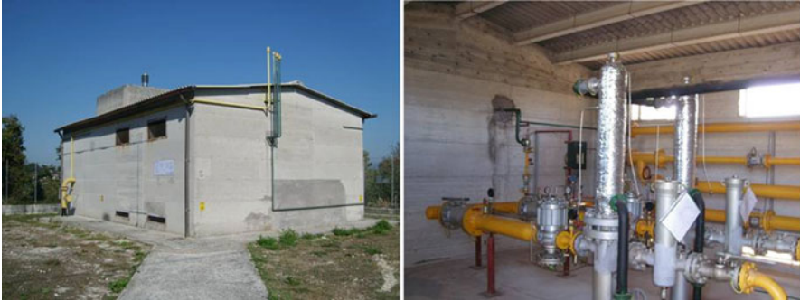
Fig. 7.1 Pictures of the outside ( left ) and inside ( right ) of a RE.MI cabin (Esposito et al. 2013)
