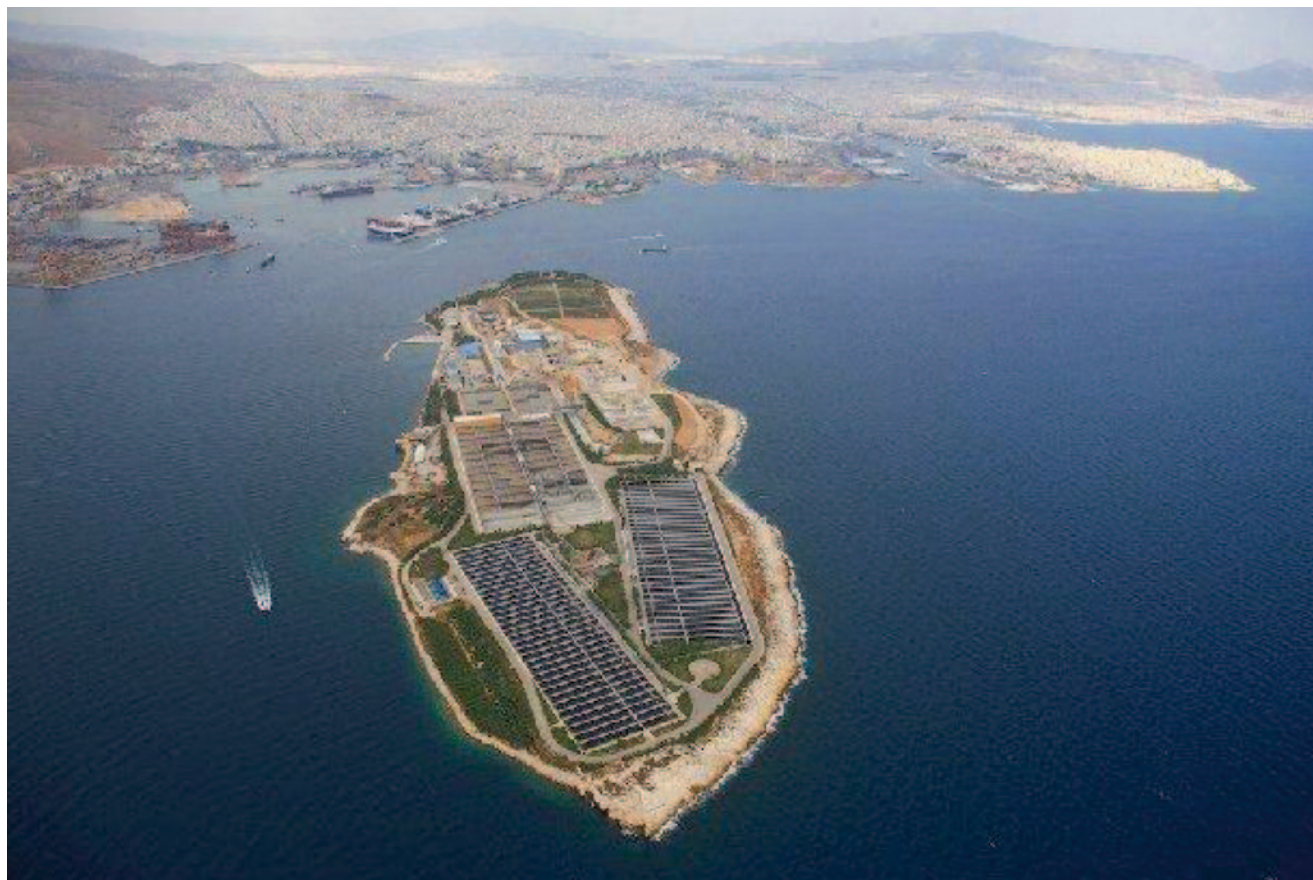
Fig. 10.1 Athens Sewage Treatment Plant in Psittalia Island
