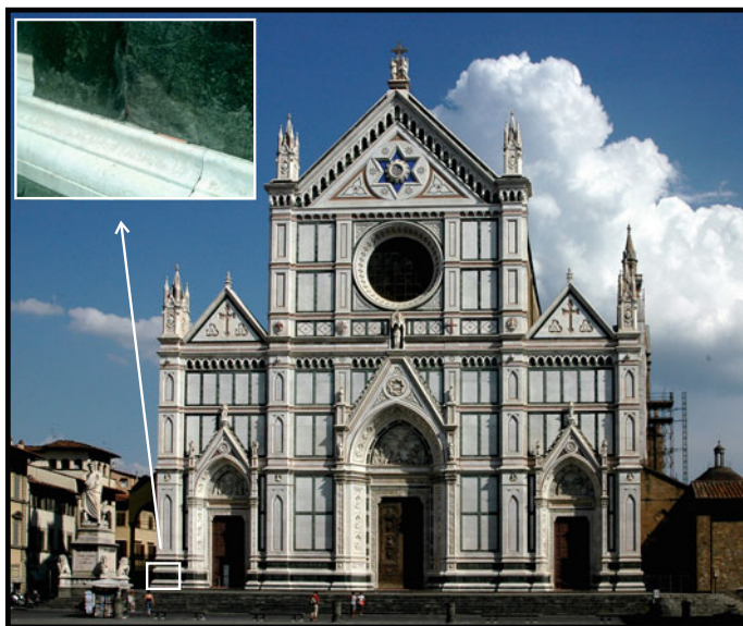
Fig. 5.7 Basilica of Santa Croce in Florence (Italy). The construction was completed in 1385. Several marble types were used in the façade: the white marble was quarried in Seravezza, and the dark serpentine marble from Pisa; the remaining marble types were quarried in other parts of Italy or imported from abroad. The inset shows the higher degree of weathering in the dark serpentine marble when compared with the white variety (Photograph by P. J. Depetris). The Basilica's image from Wikimedia Commons
