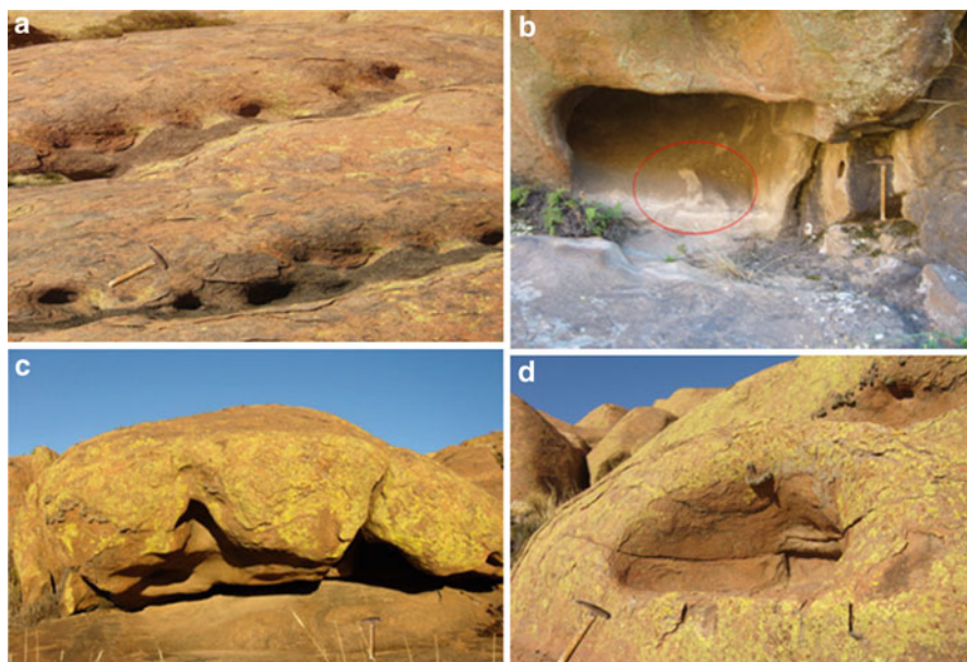
Fig. 19 (a) Tafoni appear as arranged in certain orientations, according to weakness surfaces within the ignimbrite mantles, following the boundaries in between flow units. (b) In the inner part, saline chemical precipitation is observed, in this case depicted by a red circle . (c) The inner part of the cavity is covered by alveoli, mamelonar shapes, and depressions of the scallop type. (d) Tafoni developed from fracture plane convergence
