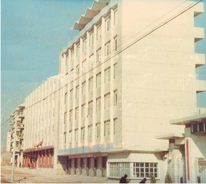
Fig. 11.3 6-storey office and retail building built with \text{Na}_2\text{SO}_4 -activated Portland-BFS-steel slag cement concrete [1]
