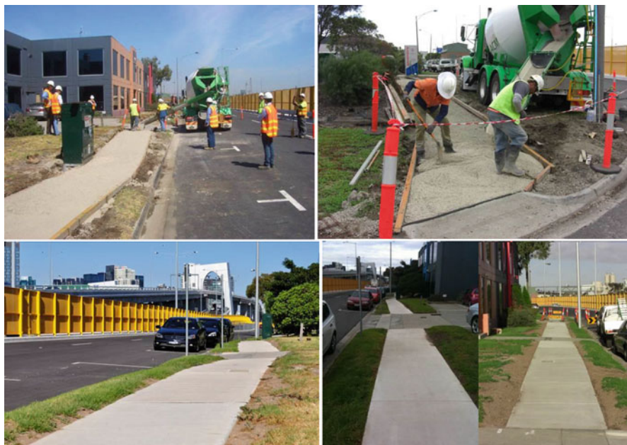
Fig. 11.18 E-Crete footpaths at Brady St in Port Melbourne, Australia
