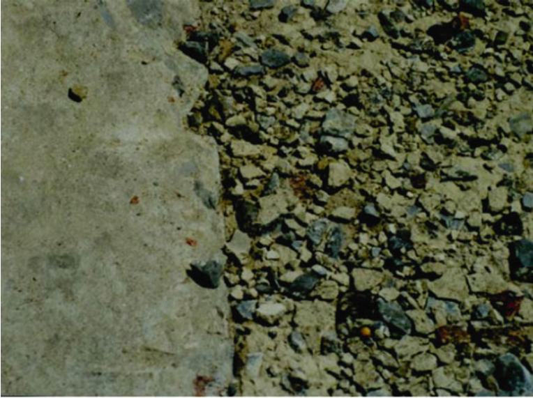
Fig. 11.5 Comparison of cast-in-situ alkali-activated slag concrete ( left side ) and ordinary Portland cement concrete road ( right ), Ternopol, Ukraine
