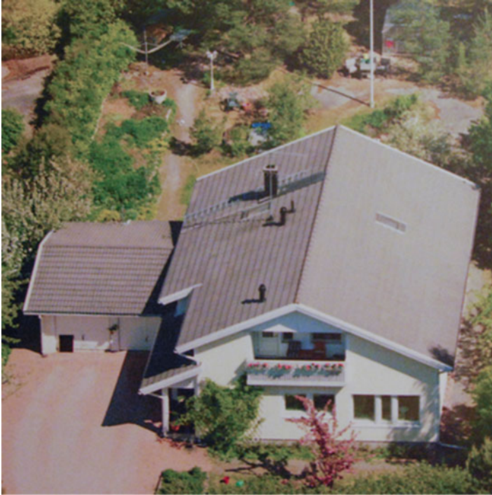
Fig. 11.8 House close to Helsinki, Finland, roofed with alkali-activated BFS tiles in 1988 (Image courtesy of B. Talling)
