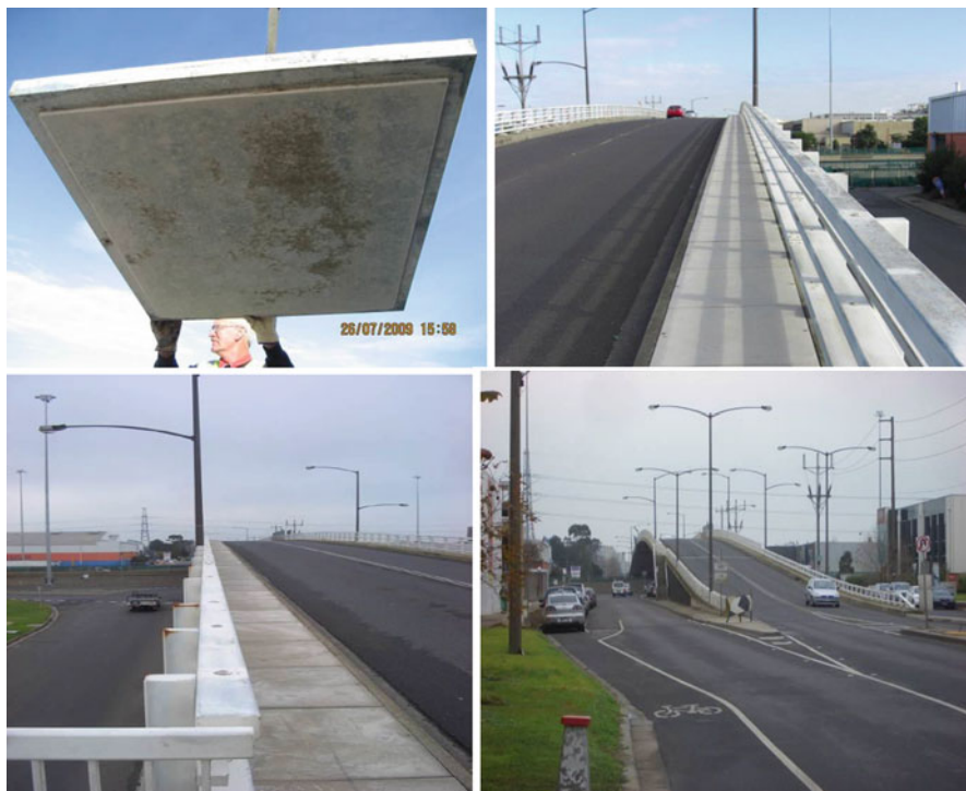
Fig. 11.16 E-Crete pre-cast footpath panel segments across the Salmon Street bridge in Port Melbourne, Australia
