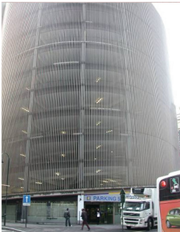
Fig. 11.7 The “Parking 58” structure, Brussels, Belgium. Parts of the first six levels were constructed from Purdociment
