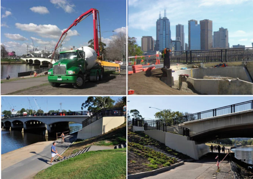
Fig. 11.17 E-Crete retaining wall at the Swan Street bridge in Melbourne, Australia
