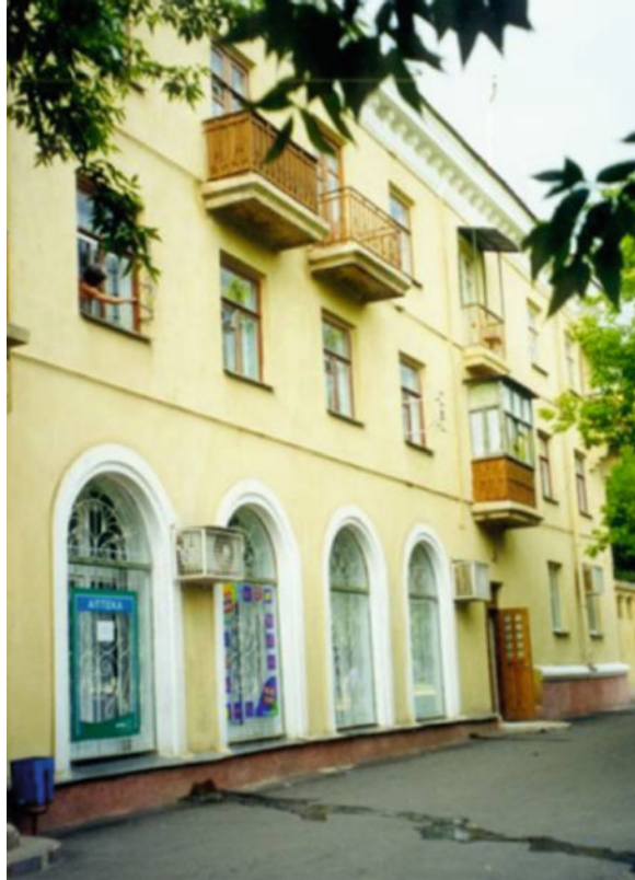
Fig. 11.2 Residential building in Mariupol, Ukraine, constructed from alkali hydroxide-activated BFS precast blocks (exterior clad in plaster) [3]
