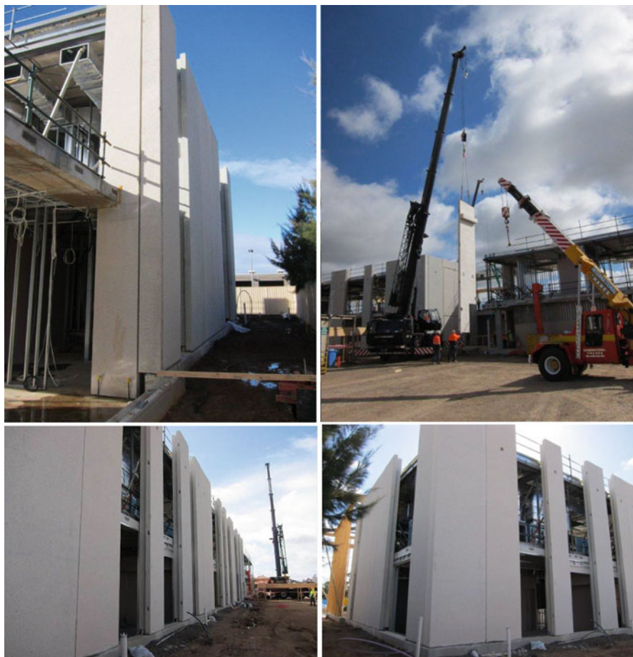
Fig. 11.20 E-Crete pre-cast panels for Melton Library, Melbourne, Australia
