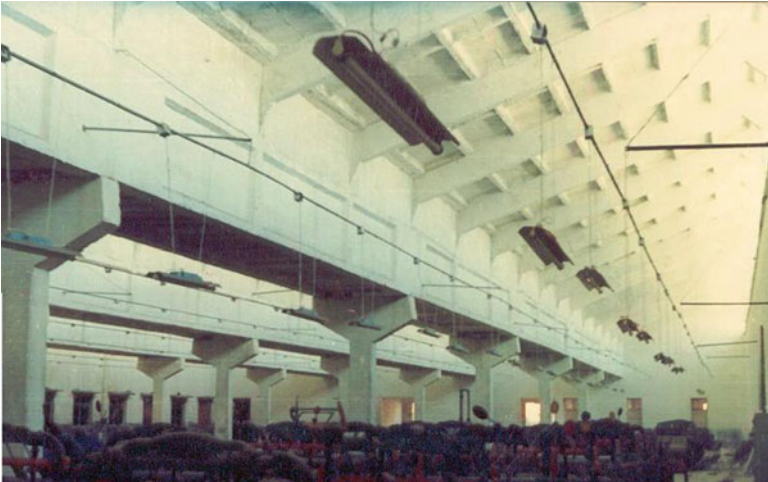
Fig. 11.4 Workshop built with \text{Na}_2\text{SO}_4 -activated Portland-BFS-steel slag cement concrete beams and columns [1]
