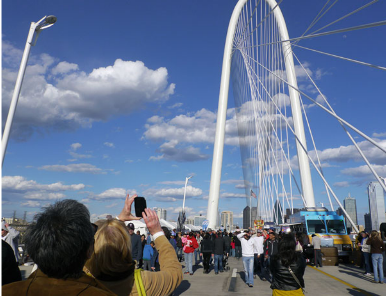
Fig. 7.4 Opening day of the Santiago Calatrava-designed bridge spanning the Trinity River in Dallas (March 2012)
