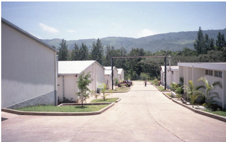
Fig. 15.7 “El Pino” rearing facility The El Pino facility (Barbarena, Guatemala) is the world’s largest fruit fly rearing facility. The four original rearing modules (at left in the picture) and two additional two-story modules provide ~10,000 m 2 of rearing area and capacity to produce >3 billion sterile male medflies per week (Image courtesy David Lance CPHST, APHIS, USDA)
