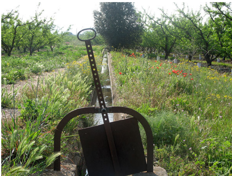
Fig. 11.4 A flooding gate (martellière), a management tool in plot farming, ASA of the Gignac Canal (Hérault) (Source: Author, 2008)
