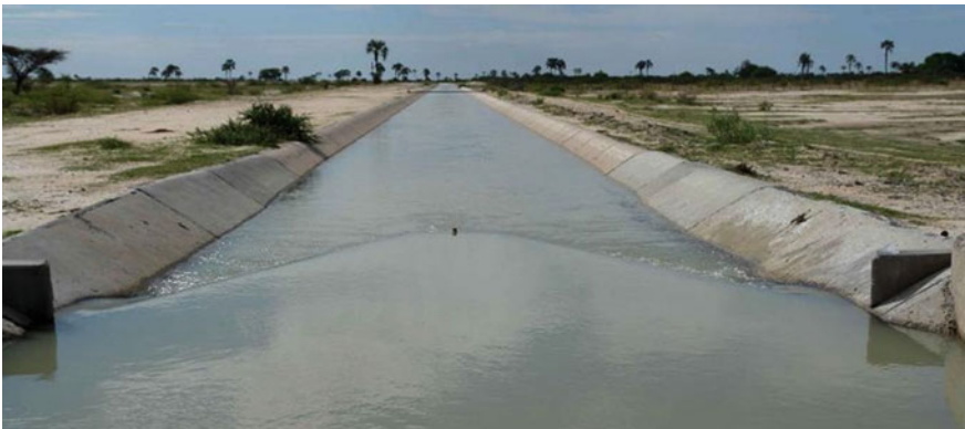
Fig. 1.3 Calueque-Oshakati canal in north-central Namibia
