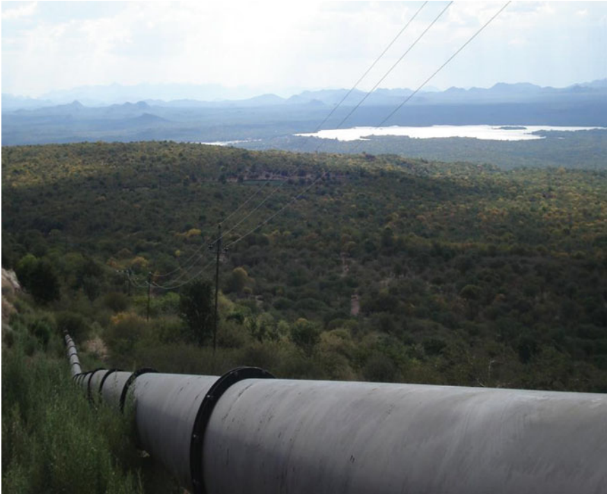
Fig. 1.2 Calueque dam and part of the Ruakana-Oshakati pipeline
