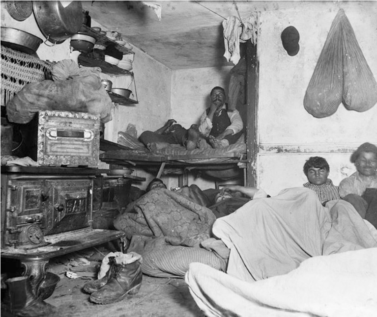
Fig. 1 “Lodgers in a crowded Bayard Street tenement” (Photograph by Jacob Riis, ca. 1890, from the collections of the Museum of the City of New York (90.13.1.158). Reproduced with permission. A sketch based on this photograph was included in Riis (1890, 69).)
