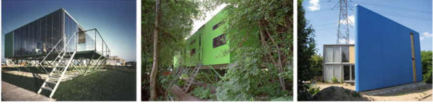
Fig. 1.7 Some of the ‘Unusual Living’ houses in De Fantasia: Hard Glas (left two images), and Blue House (right)
