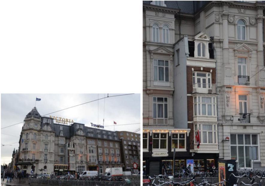
Fig. 1.1 The two small buildings, encapsulated by the Victoria hotel, Amsterdam (Photos: © Rob Roggema)
