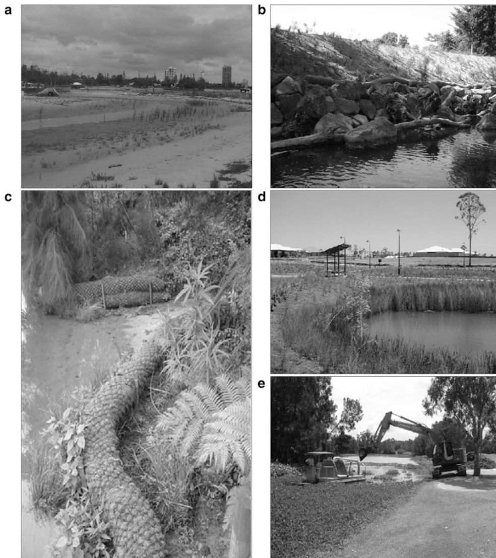
Fig. 7 Example restoration projects for the Gold Coast Broadwater and catchment waterways; (a) recolonisation of mangrove community at land reclamation beach area; (b) restoration of reach along local waterway in the city; (c) stabilisation project using soft engineering
