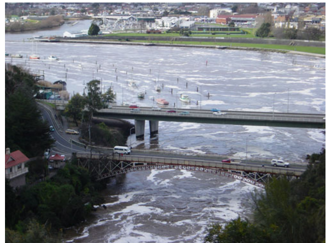
Fig. 11 The South Esk River in flood entering Home Reach at Launceston, where an arcuate concrete wall diverts flow towards the left (north) and away from Launceston in the background (Photograph: C. Shepherd)
