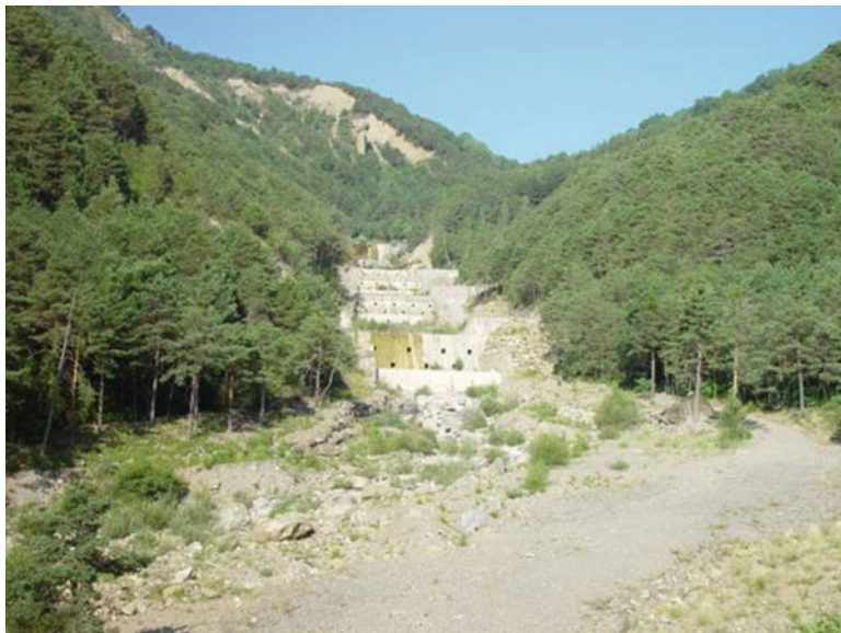
Fig. 11.6 Series of check dams at the Barranco de Arás, Central Pyrénées, Spain (© J. Corominas)
