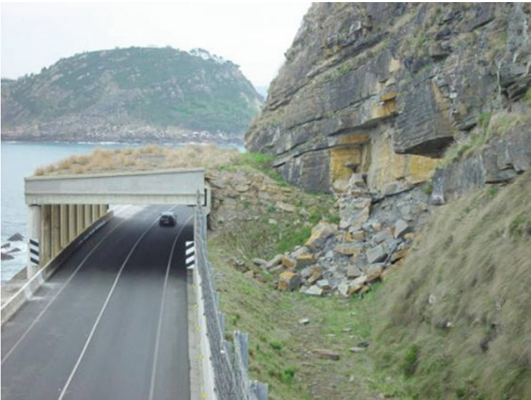
Fig. 11.5 Gallery and a combination of ditch and barrier to protect against the occurrence of rockfalls in the coastal road of Gipuzkoa, Basque Country, Northern Spain (© J. Corominas)
