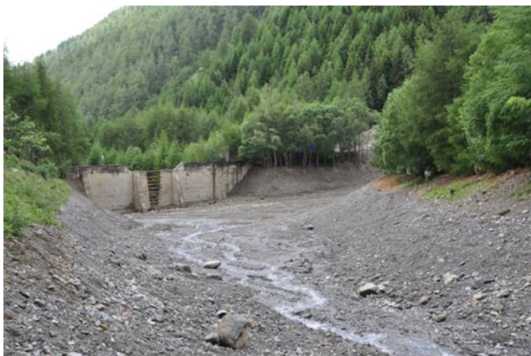
Fig. 11.7 Retention basin, Bolzano Province, Italy (© J. Corominas)
