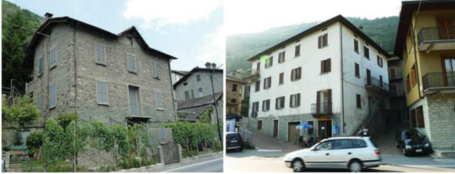
Fig. 14.3 Typical stone wall ( left ) and brick masonry ( right ) houses in Tresenda
