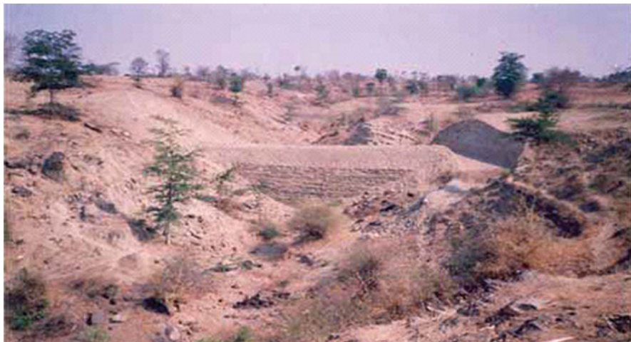
Fig. 14.3 Severe gulying may require structural works to reduce flow and trap sediment
