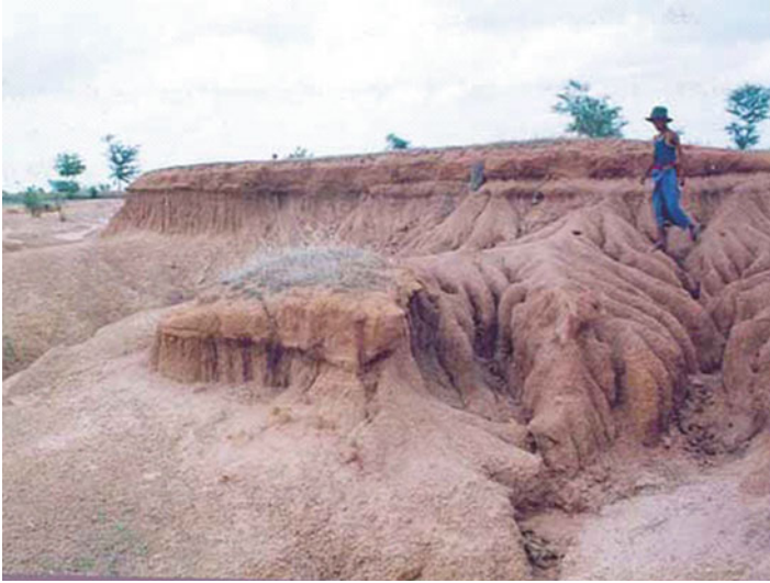
Fig. 14.2 Severe gullying and soil loss can follow deforestation and inappropriate cultivation methods
