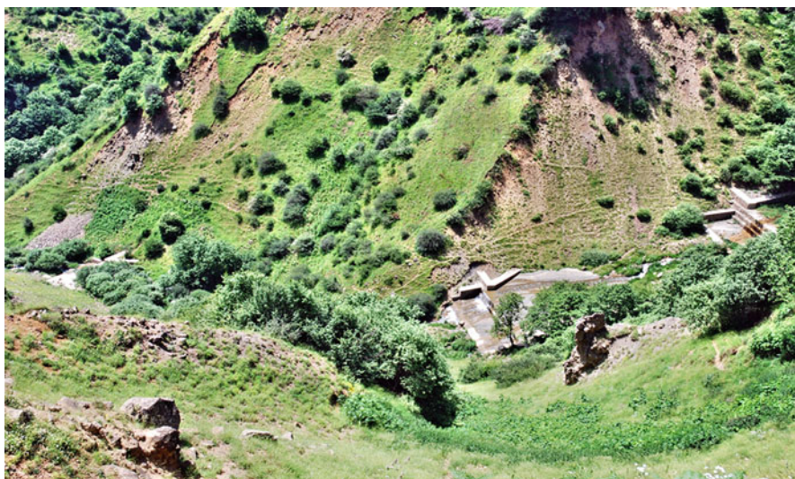
Fig. 14.4 Structural gully control works are an effective means for control of sediment movement
