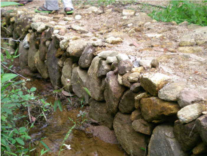
Fig. 16.13 Stone walls were built by the local community to combat erosion
