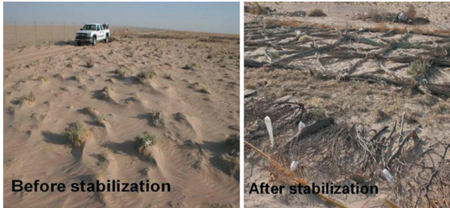
Fig. 19.3 Low cost materials (palm fronds and other debris) have been used to stabilize sandy areas and reduce the impact of dust and sand storms
