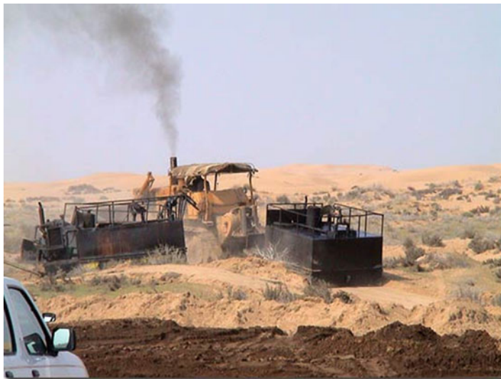
Fig. 17.7 Bulldozer towing oil/seed spraying equipment into position
