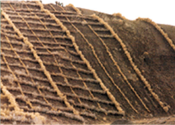
Fig. 17.6 Prevention of the wind erosion can be achieved by covering the surface with obstacles that reduce wind velocity at the surface
