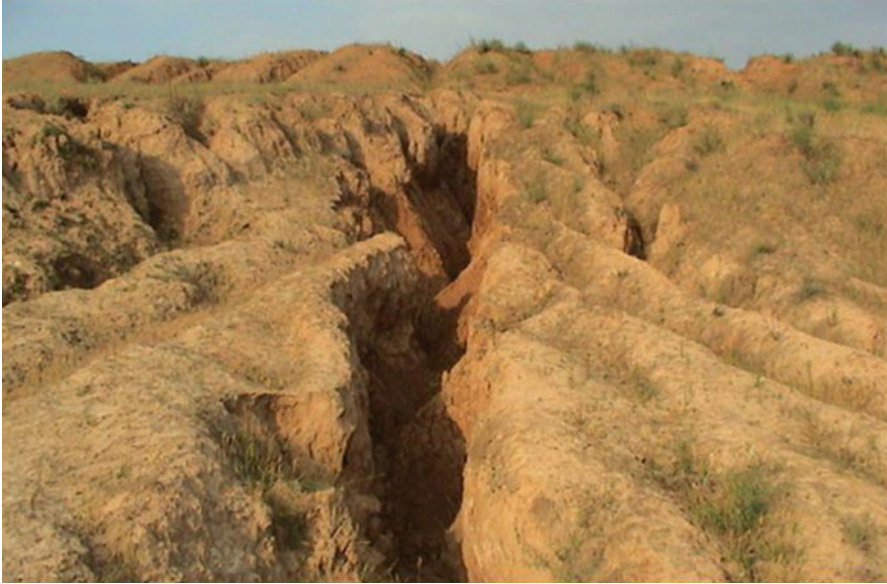
Fig. 18.3 Severe gully erosion in loess area
