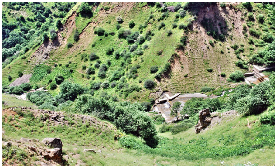
Fig. 14.4 Structural gully control works are an effective means for control of sediment movement
