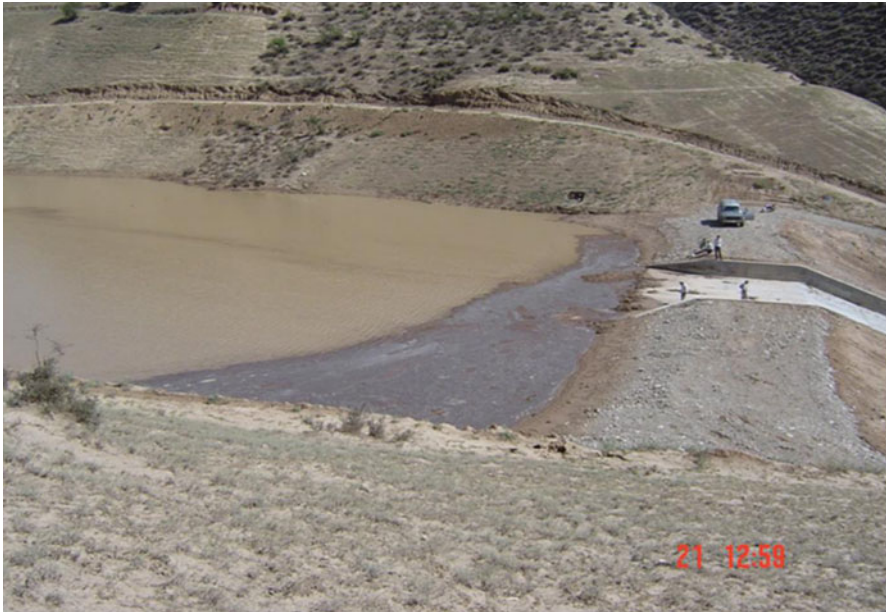
Fig. 18.7 Small dams allow water harvesting and assist in flood mitigation in an upland catchment of Atrak river
