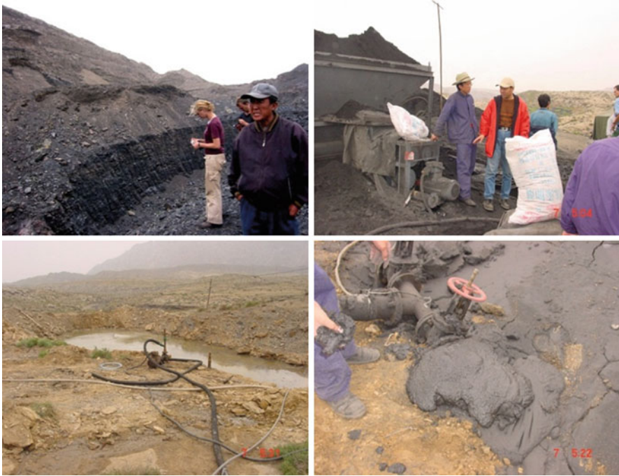
Fig. 21.3 Examples of coal fire extinguishing attempts. Upper left: on the upper left part of the image can be seen former mine entrances, which were improperly sealed with loess and sand. The coal seam below is burning. To rescue other parts of the seam from igniting as well (the part where the people are located), a trench was dug by local miners to separate the burning part of the seam from the not (yet) burning part. The other three photographs show the attempt to pump a mixture of water, coal dust, ash, and special colloids into the underground to fill up cavities and cracks and therefore deplete the fire of oxygen (Photographs taken in Wuda, China, by J. Zhang)
