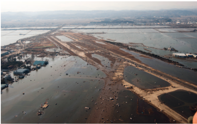
Fig. 4.12 Sendai airport on March 16, 2011 flooded with water inundation due to the tsunami
