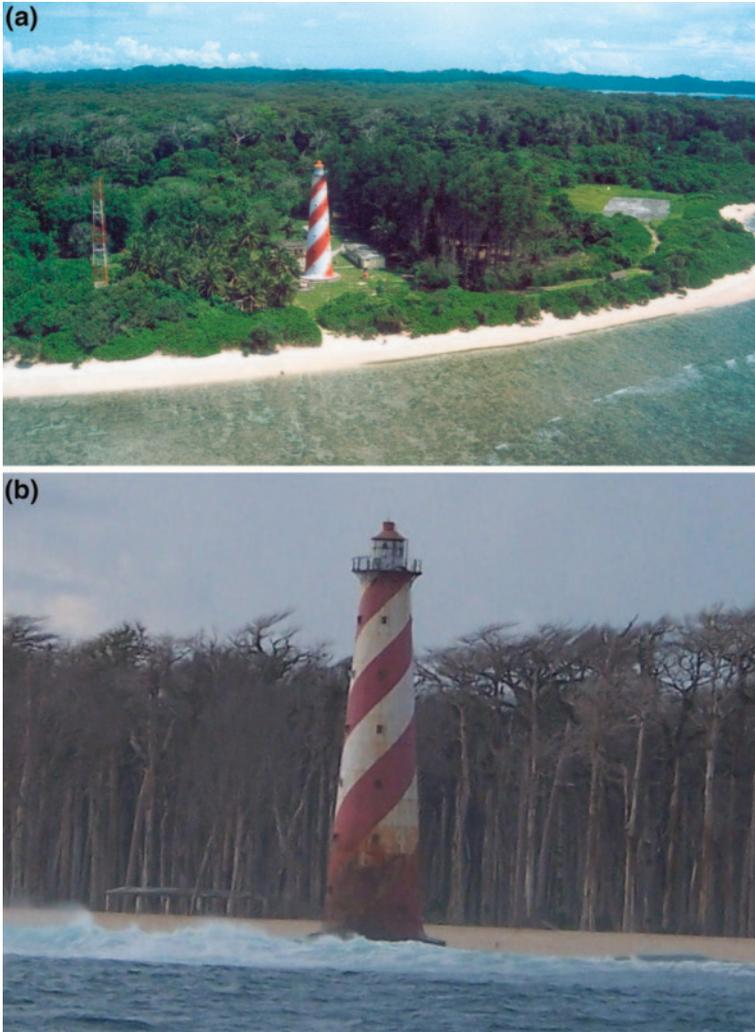
**Fig. 3.14** A photo combo of the light house at Indira point at Great Nicobar Island before and after the earthquake. Coseismic subsidence of more than 1 m and extreme inundation due to the tsunami can be seen here
