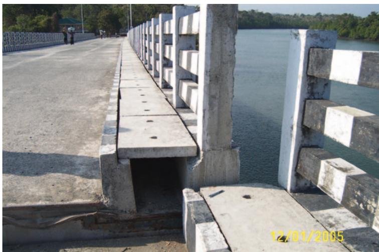
**Fig. 3.12** The Ashton creek bridge in North Andaman was offset by more than a foot by extensive ground shaking
