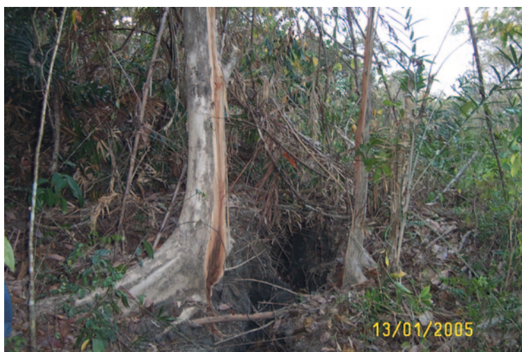
Fig. 3.16 There were large cracks in the mud-volcano region and in one case, the trunk of a tree got split
