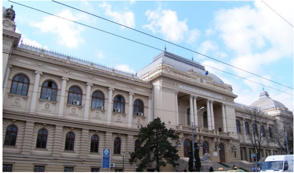
Fig. 22 View of Palace of “Alexandru Ioan Cuza” University of Iasi which was constructed in two stages: first in 1894 and then in 1928–1934
