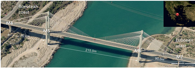
Fig. 1 The central section of the Evripos cable-stayed bridge
