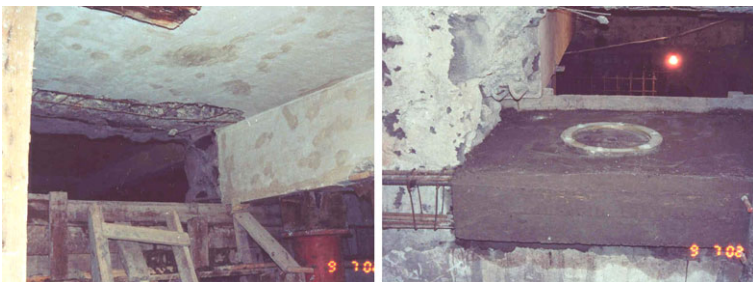
Fig. 12 Existing beam is crossing the space of the opening and supported by temporary columns
