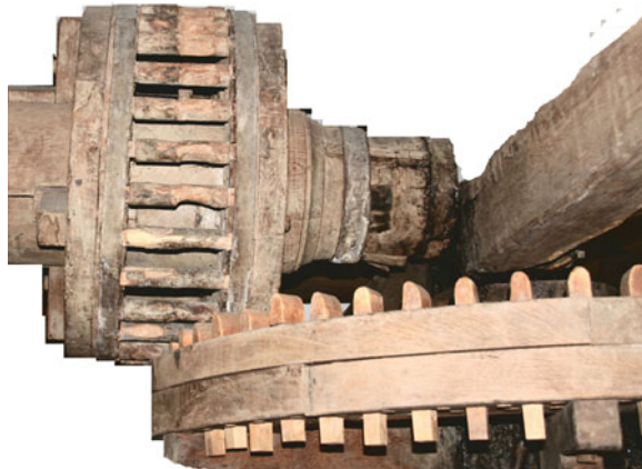
Fig. 6 Design and appearance of wooden gears after many years of in operation
