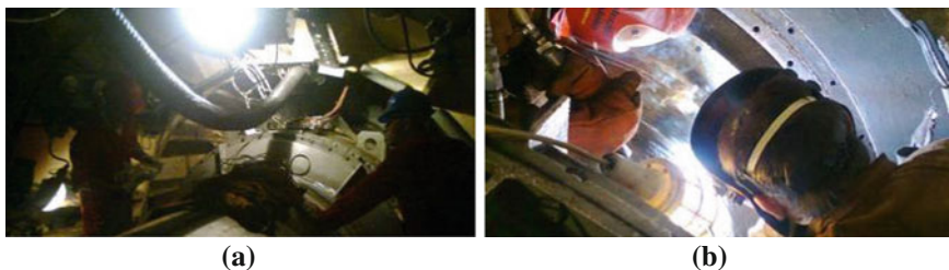
Fig. 9 Presentation of limited space for the shaft recovery. a Shaft prepared for recovery. b Position of the welding operator during recovery
