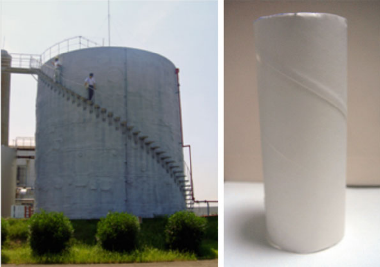
Fig. 7.4 A toilet paper tube as a similar model for the spiral banister of an oil tank
