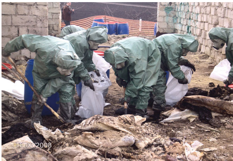
Fig. 38.3 Cleaning of an abandoned obsolete pesticide storage site
