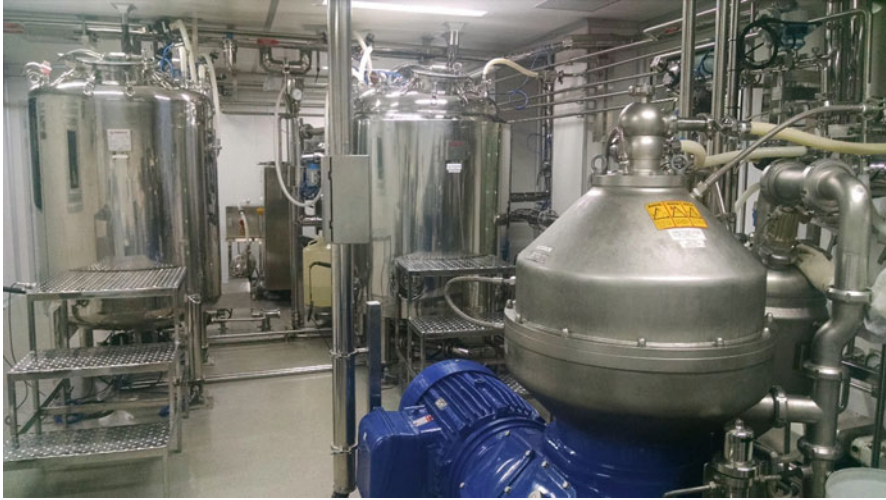
Fig. 1 Enclosed and automated purification plant of Instituto Butantan, showing the fractionation tanks and the ultracentrifuge used in the process of antivenom production
