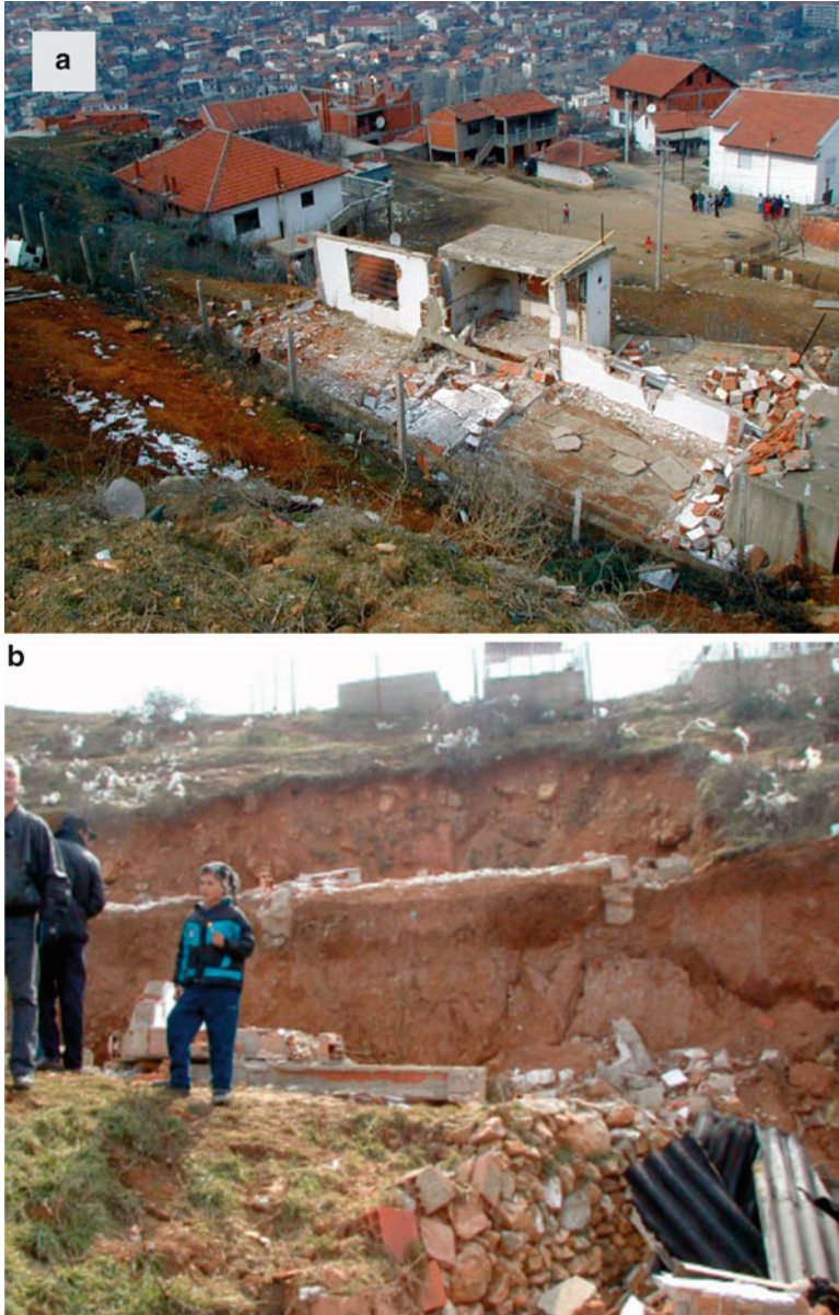
Fig. 17.4 View from the top of the Ramina landslide onto the built-up area (a) and on the main scarp (b) (Photos by M. Jovanovski)
