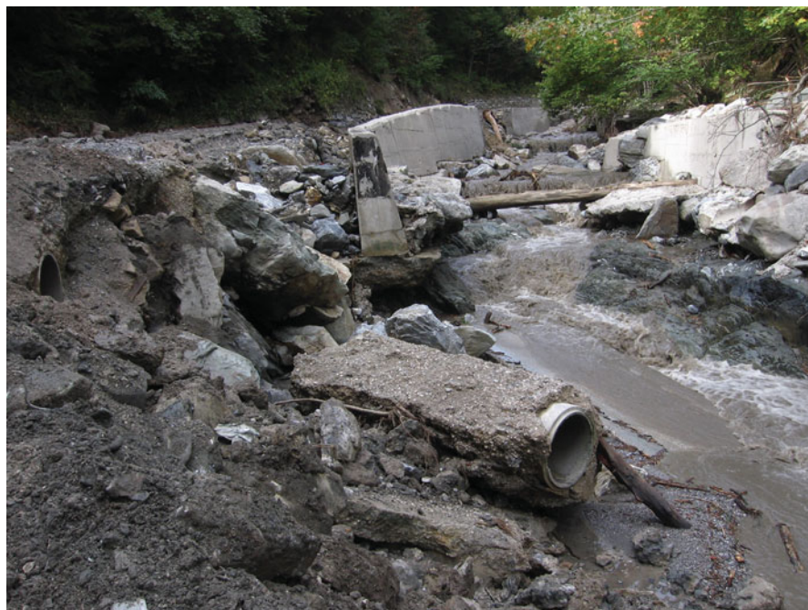
Fig. 8.4 Consequences of flash floods in the Davča Valley (western Slovenia) during the 2007 floods (photo by M. Zorn)
