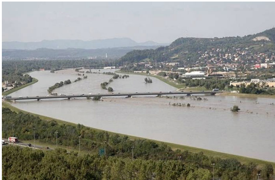
Fig. 9.2 The Sava at its entrance into Zagreb, 19 September 2010 ( Source: Hrvatske vode)
