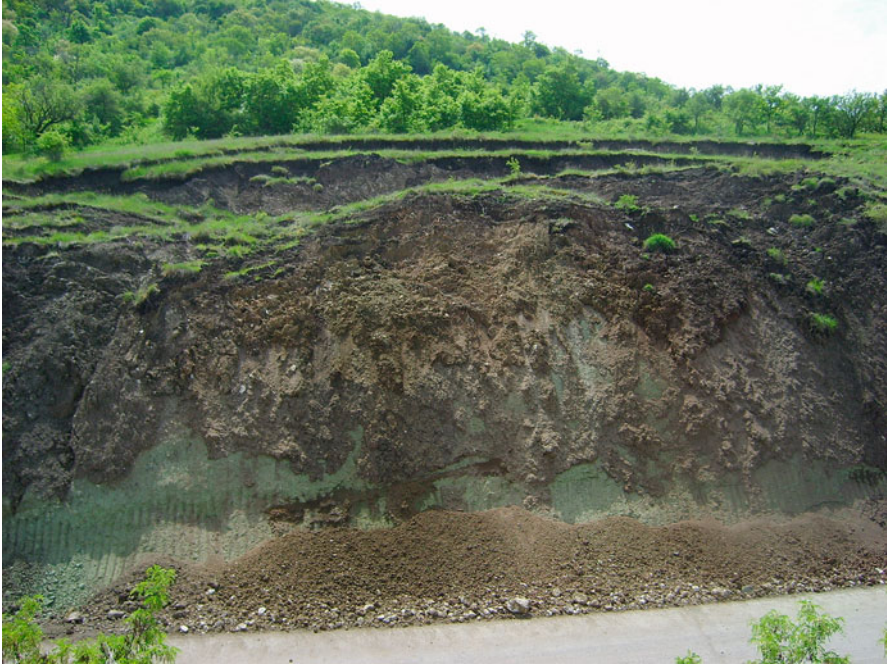
Fig. 17.9 The Stracin landslide on the international road Corridor 8, highly active in early 2010 (Photo by I. Milevski)
