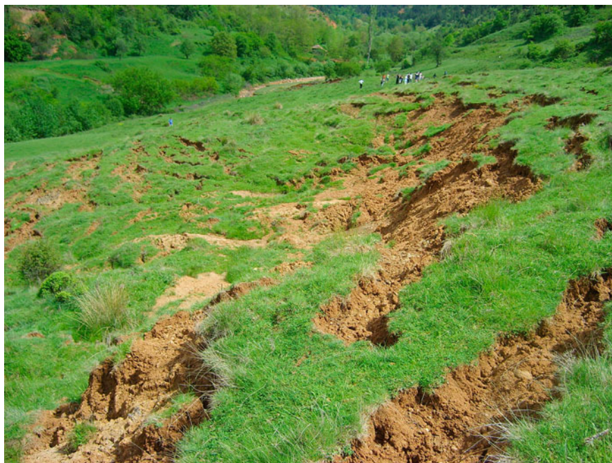
Fig. 17.8 Cracks on the Crnik landslide and mass movement towards the Crnička River in May 2010 (Photo by I. Milevski)
