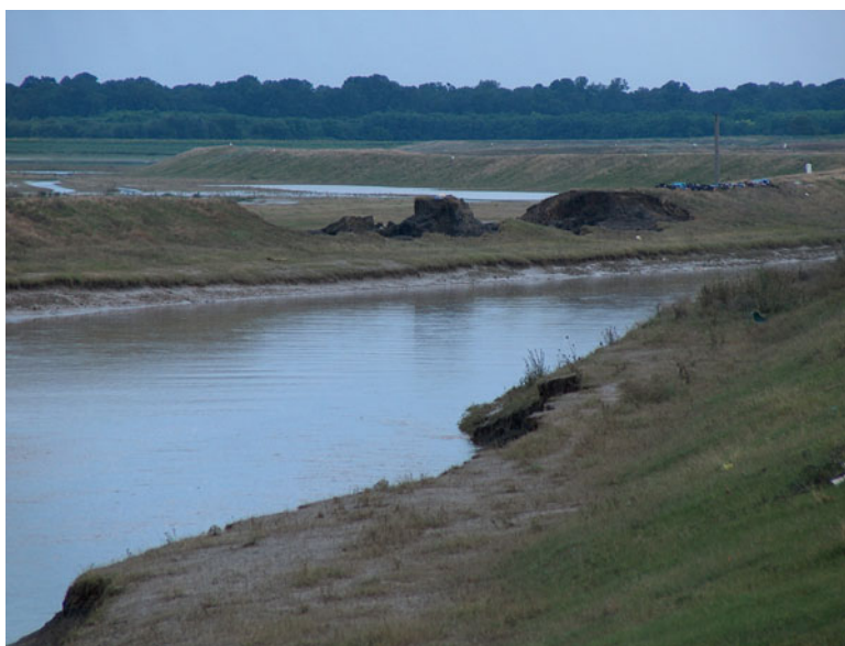
Fig. 7.2 Dam breach at Condrea village
