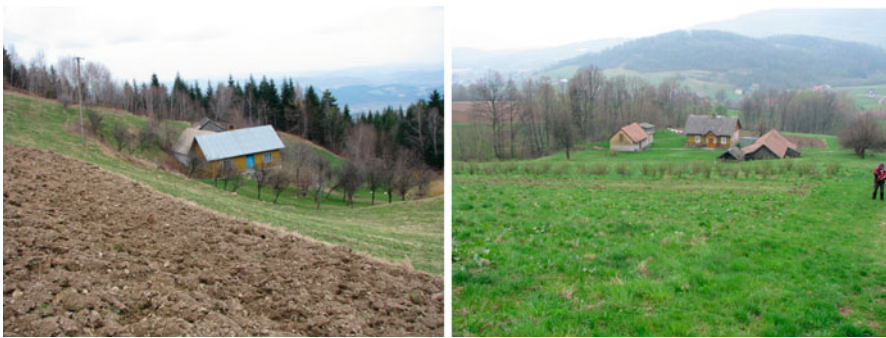
Fig. 15.5 Examples of houses located in landslide niches
