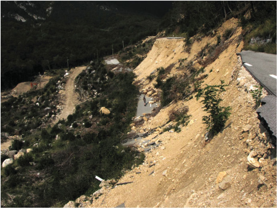
Fig. 8.7 During extensive precipitation in September 2010, the Stogovce landslide was triggered, which destroyed a kilometer of the road between Ajdovščina and Predmeja (photo by M. Zorn)
