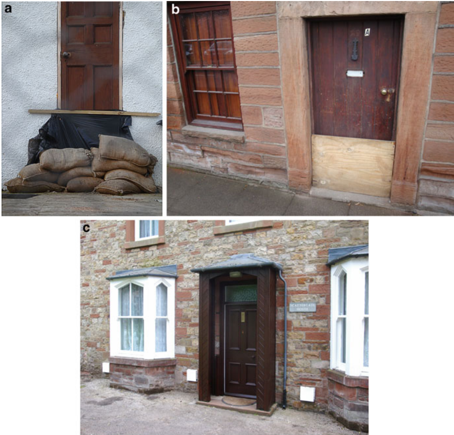
Fig. 4.1 Examples of flood barriers: (a) sandbags; (b) a home-made door-board made of marine ply, and (c) commercially available airbrick covers ( Source: The author)
