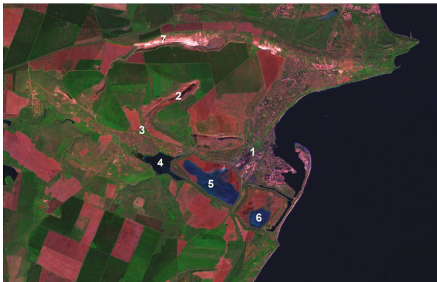
Fig. 27.1 Main geomining objects in Kerch district. Legend: 1 iron ore agglomeration plant, 2 iron ore open cast quarry, 3 Churbash ravine, 4 Churbash Lake, 5 and 6 iron ore waste depository, 7 limestone quarry (see color plates)
