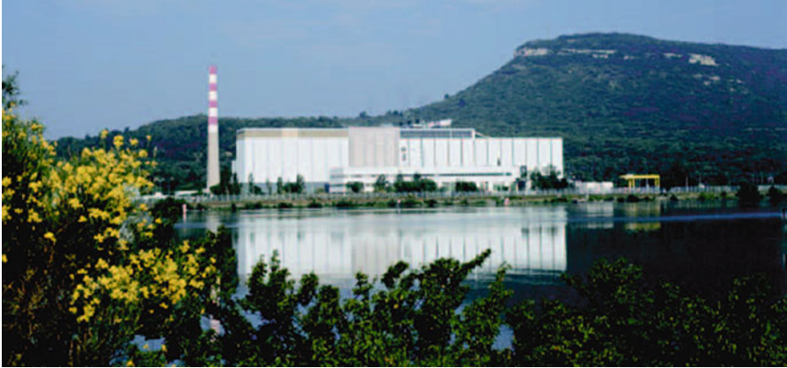
Fig. 7.2 Phénix sodium-cooled fast-neutron reactor in Marcoule (France) ( see color plates )
