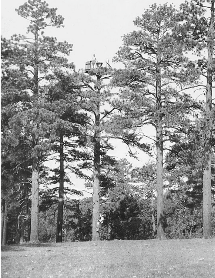
Fig. 1.30 Lookout tree in Kaibab National Forest, north-central Arizona. Trees were used to locate fires for suppression before fire lookout towers were built. Note person on platform at top of tree about 19 m (62 ft) above the ground and person climbing ladder attached to tree. Information in National Park Service (1987) suggested undated photograph is possibly from 1916 (Photograph by U.S. Forest Service, Southwestern Region, Kaibab National Forest)
