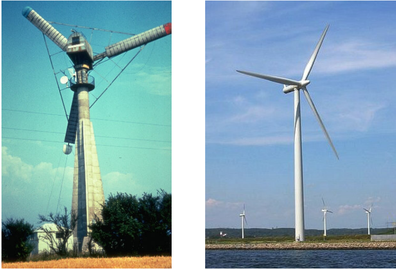
Fig. 2 Left figure: The 200 kW Gedser wind turbine erected in 1957; Right figure: Modern 2.5 MW wind turbine
