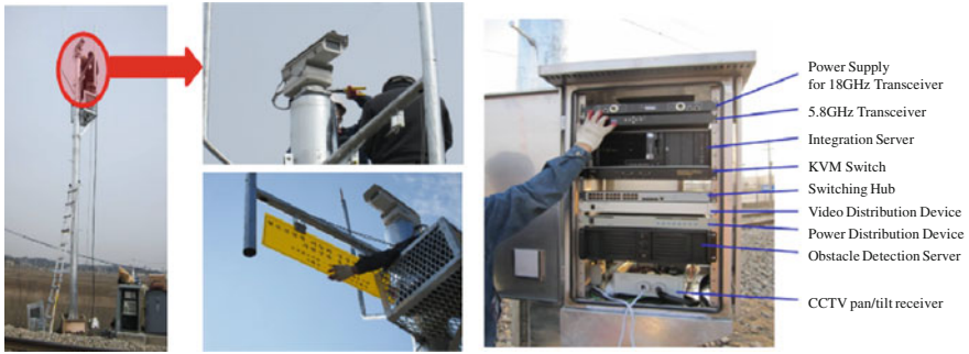
Fig. 3 Installation of CCTV camera and control cabinet
