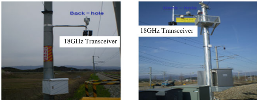
Fig. 4 Installation of bidirectional wireless transceiver
