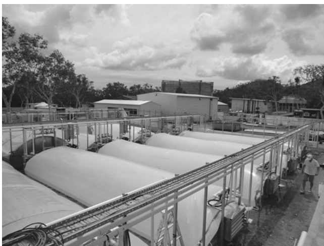
Fig. 7.9 Biological Algae Growth Systems (BAGS) developed by MBD Energy Ltd (Australia) (Courtesy of MBD Energy Ltd)
