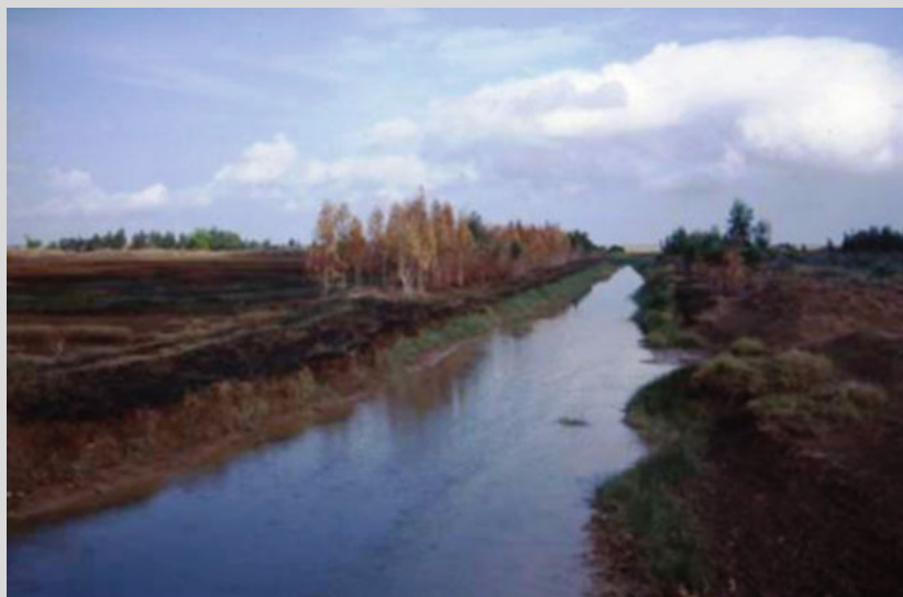
Fig. 13.2 Drainage canals constructed in the Melaleuca forest for access and to drain the swamp to allow agricultural development (Photo Peter Burbridge)
