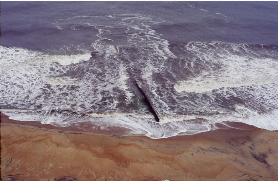
Fig. 26.8 A rip current is generated by a groin at Cape Hatteras, North Carolina (Source: S. P. Leatherman)
