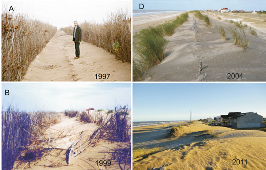
Fig. 19.22 Dune reconstruction in San Clemente del Tuyú between 1997 and 2004, Buenos Aires. (a) Barrier fences installation; (b) Sand deposition after 2 years; (c) S. coarctata plantation; (d) Current view
