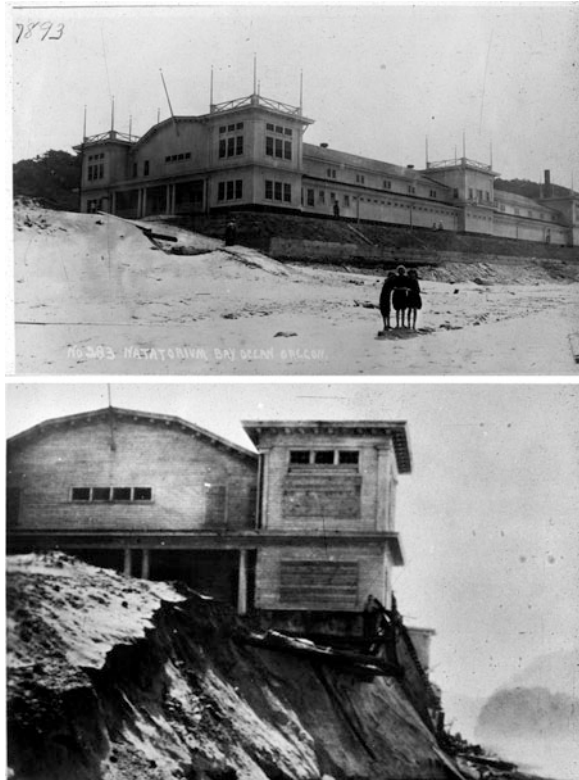
Fig. 21.11 Progressive loss of the Natatorium (containing an indoor swimming pool) on Bayocean Spit: ( Top ) from 1910 and ( Bottom ) in 1932 after a jetty had been constructed on the inlet to Tillamook Bay (Courtesy of the Pioneer Museum, Tillamook, Oregon)
