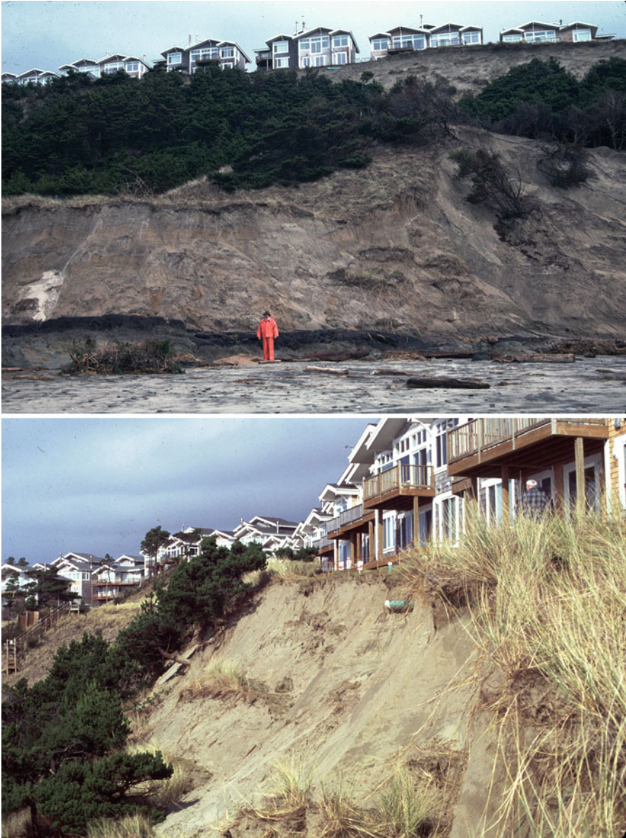
Fig. 21.18 The Capes development of condominiums north of the inlet to Netarts Bay located on an old landslide: ( Upper ) Toe erosion during the 1997–1998 El Niño, having reactivated movement of the slide; ( Lower ) The first line of condos being threatened by the slip-face of landslide movement (From Komar (1998a))
