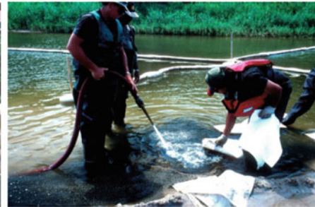
Ground view of sand flushing to remove oil within pore spaces of the sand bar pictured to left (Swanson Creek spill, Maryland, USA),
