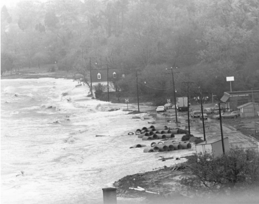
Fig. 13.32 Yorktown during a storm in 1978 prior to headland beach installation (Photograph courtesy of Scott Hardaway)
