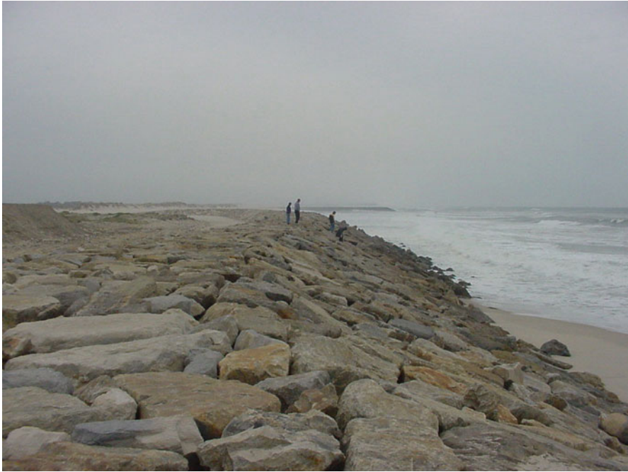
Fig. 17.11 Sea wall protection in north Portugal
