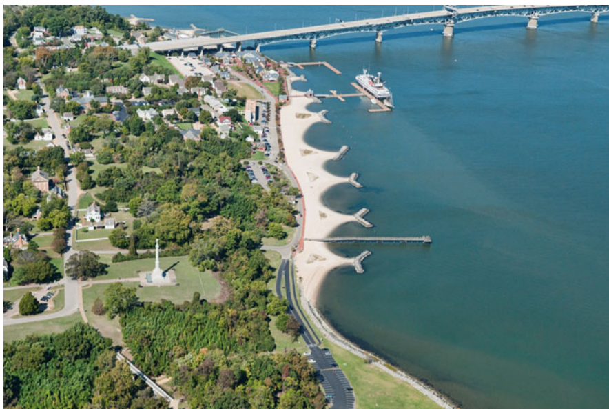
Fig. 13.33 Photograph of the headland beach system constructed on the south side of Yorktown River. Portions of this installation had been in place for 18 years as of 2012 and were undamaged by Hurricane Isabel in 2003 (Photograph courtesy of Scott Hardaway)
