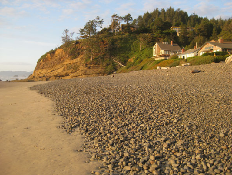
Fig. 21.10 The Composite Beach at Oceanside on the northern Oregon coast, offering protection to the vegetated sea cliff along that community (Photo J.C. Allan)
